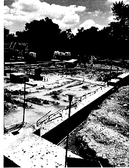
2018.06.28 – Foundation stems walls have been installed at the main entry.
