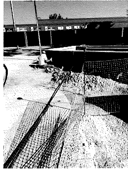
2018.07.16 – A worker is removing the waterproofing overspray from the site walls.
