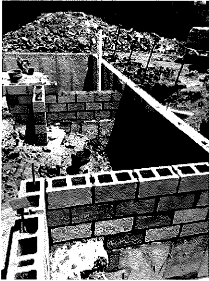
2018.06.28 – Installation of the concrete masonry walls has begun.
