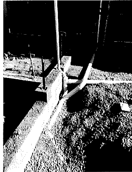
2018.07.16 – Installation of the under-slab plumbing in the mechanical room is in progress.
