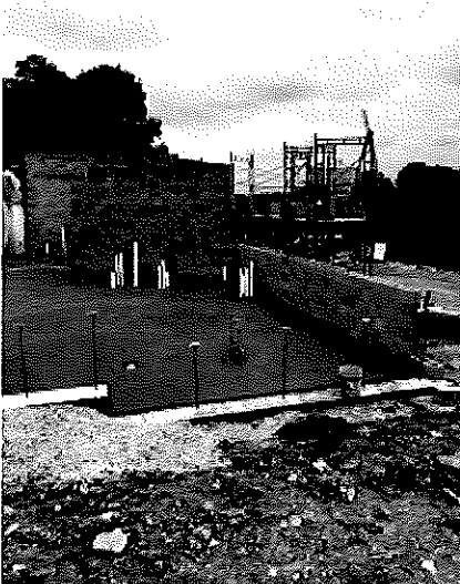
2018.07.23 – The slab-on-grade has been poured and is being finished.
