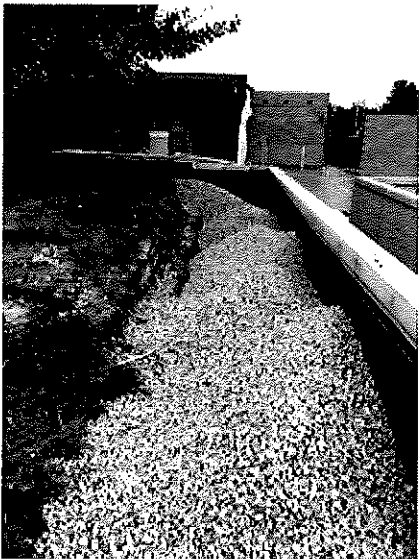
2018.07.23 – The site walls have been backfilled with self-draining granular fill.
