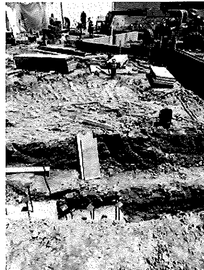
2018.06.28 – Formwork is being installed for the foundation stem walls.
