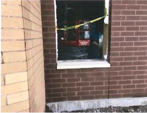
2016.12.05 – Cast sill in place.
