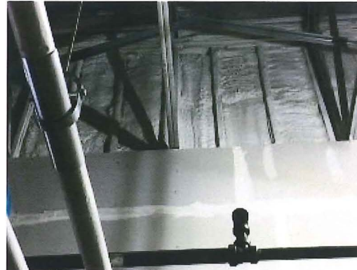
2016.12.08 – Spray foam insulation at truss end wall.
