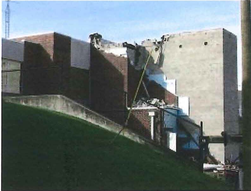
2016.12.05 – Demolition of existing stair tower.
