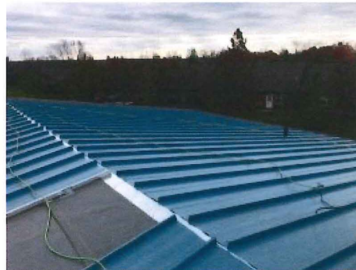
2016.12.01 – Metal roof installation
