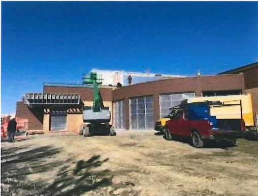
2016.12.08 – Weather enclosure and crew working at platform enclosure above.
