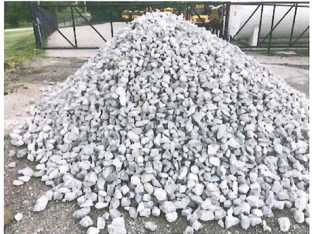
2018.06.11 – gravel for south construction entrance
