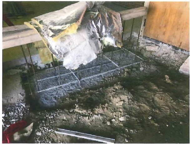
2018.06.19 – Footing at firewall portal frame
