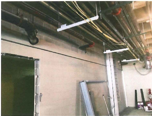
2018.06.19 – New hangers along east end of firewall
