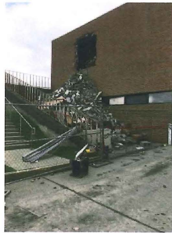
2018.06.12 – Dumping debris out a wall opening at the upper level
