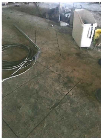
2018.06.19 – Saw cut for plumbing trench
