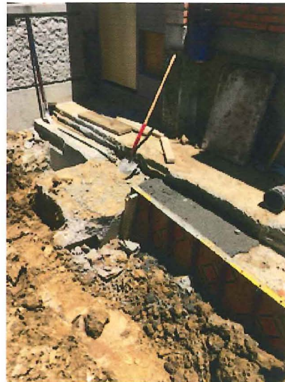
2018.06.04 – Underpinning outside Room No. 113 and 114 is in progress.
