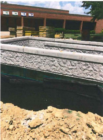
2018.06.18 – Waterproofing and protection board has been installed on the exterior site and ramp walls. Where the material is too high it will be cleaned off.
