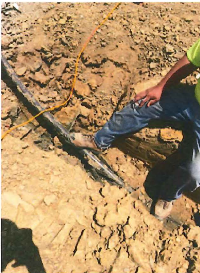
2018.06.18 – An abandoned underground electrical cable was discovered.
