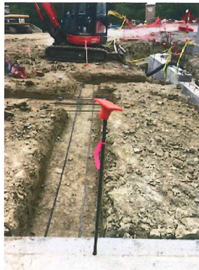
2018.06.18 – Installation of the building footings and stem walls for the new addition has started.
