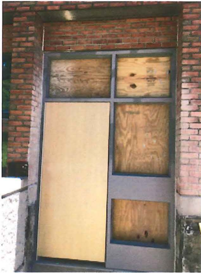
2018.06.04 – The door frame for the temporary exit from Room No. 114 has been installed.
