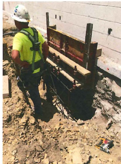
2018.06.18 – Underpinning of the existing building wall is in progress.
