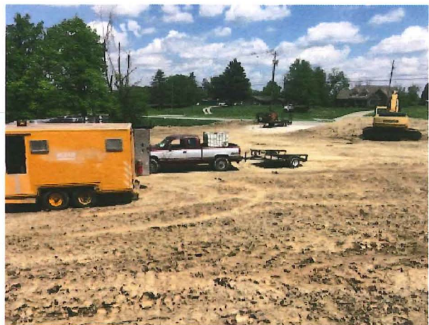
2018.05.10 – Grading at well field
