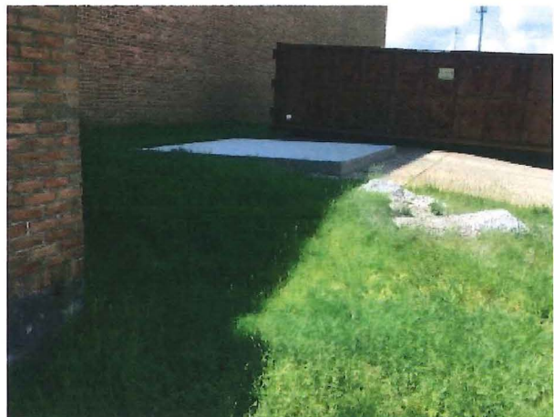
2018.05.10 – Leveling slab for relocated Beechgrove cooling tower.
