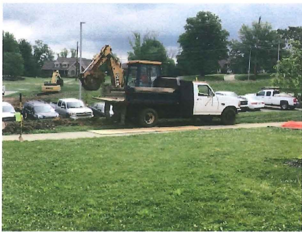
2018.05.22 – Excavating for new fire/water service vault
