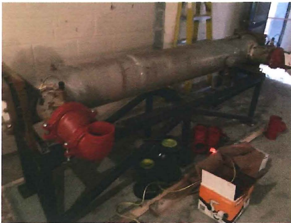
2018.05.22 – Temporary barrel chiller
