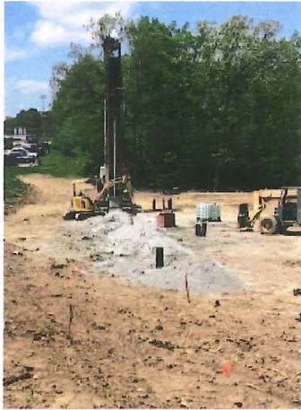
2018.05.10 – Drilling geothermal well
