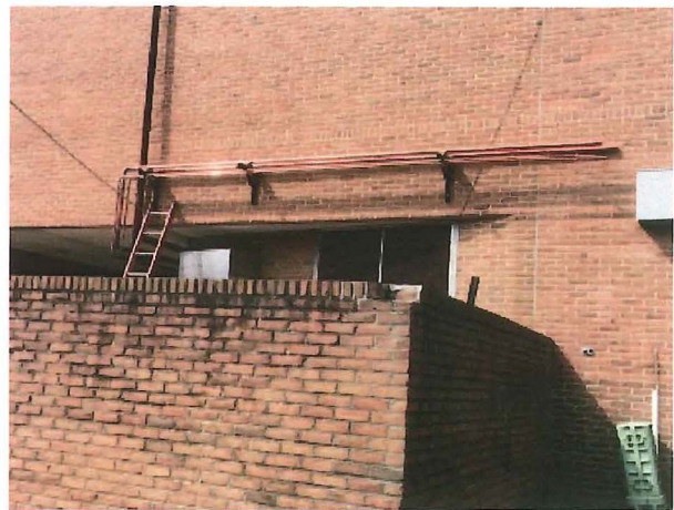
2018.05.22 – Temporary chiller piping
