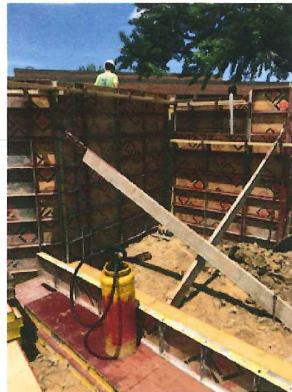
2018.05.021 – Construction of the form work for the new ramp and stairs is in progress.
