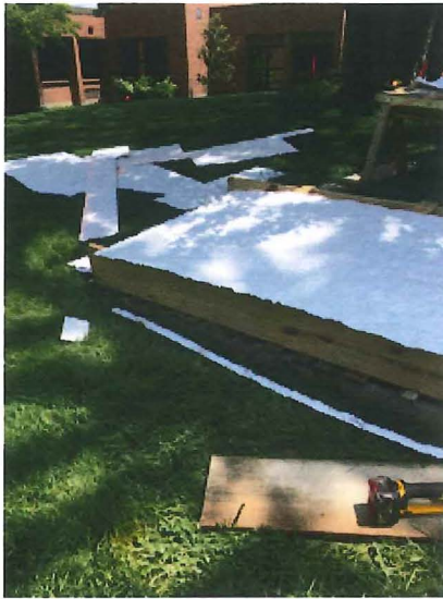
2018.05.21 – Formliners for the textured walls on the new ramp and exterior stairs.
