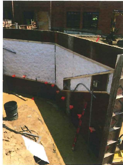
2018.05.21 – Construction of the form work for the new ramp and stairs is in progress.
