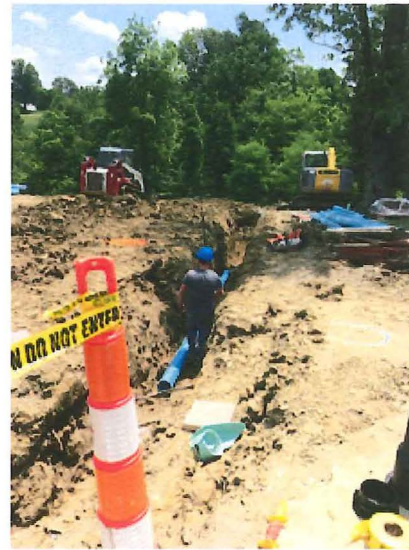
2018.05.21 – Installation of the re-routed sprinkler main to the south of the building is in progress.
