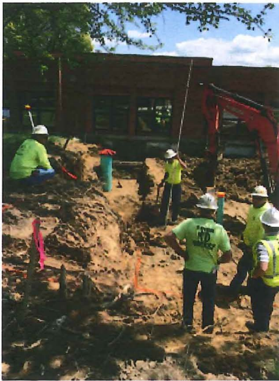
2018.05.07 – Excavation for the footings for the new ramp and stair is in progress.
