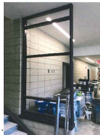
2018.05.10 – guard awaiting infill panels
