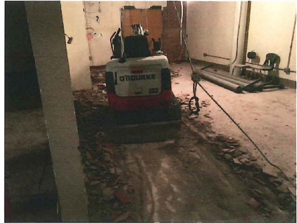
2018.04.23 – Quarry tile removal in former serving.
