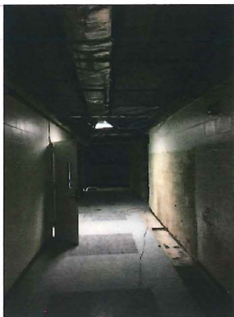
2018.04.23 – Ceiling removed in existing corridor.
