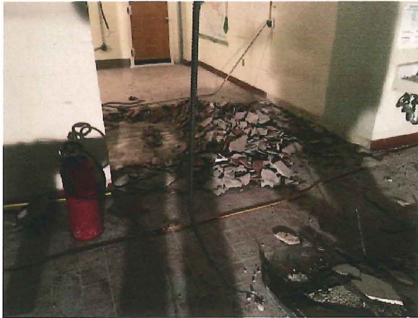
2018.04.23 – Quarry tile removal in former kitchen.
