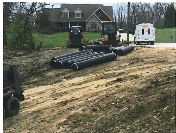
2018.04.23 – Storm piping staged for installation.
