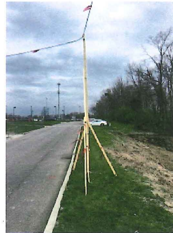
2018.04.23 – Temporary electric to trailer.
