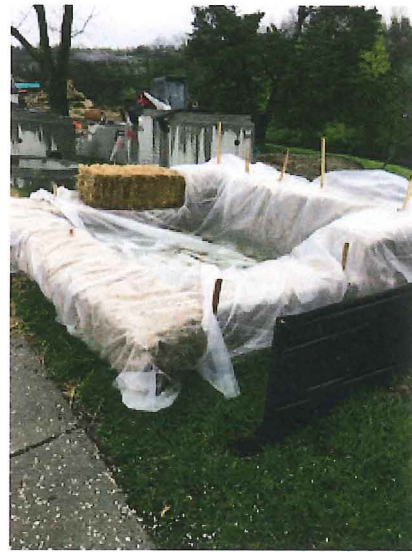
2018.04.24 – Concrete wash-out area has been set up.
