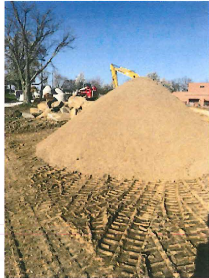
2018.04.12 – Sand for backfilling around the storm structures has been stockpiled.
