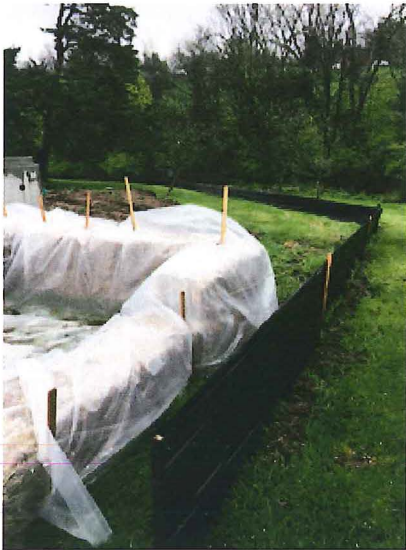
2018.04.24 – Silt fence has been installed around the perimeter.
