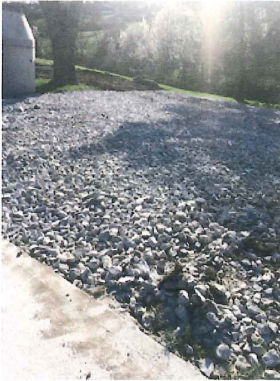
2018.04.12 – Laydown area has been graveled.
