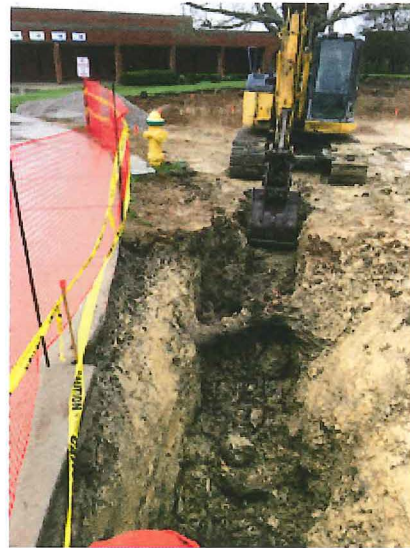
2018.04.24 – Installation of the underground storm structures has begun.
