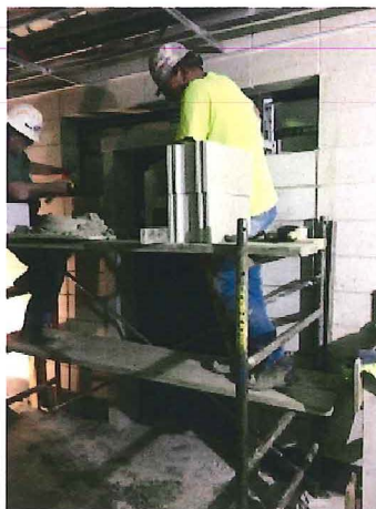
2018.04.12 – Masons infilling around elevator door.
