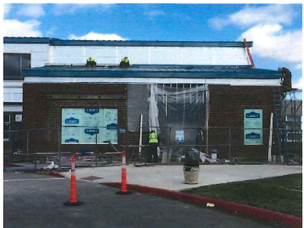
2018.01.30 – Metal installer working on base of wall flashing.
