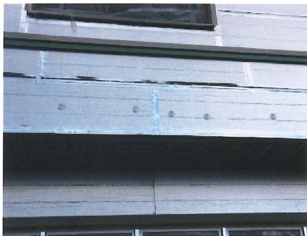
2018.01.30 – Example of taped joint needing correction.
