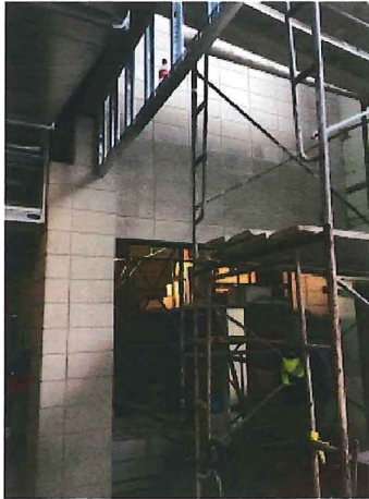
2018.01.30 – Bulkhead framing at entry interior.
