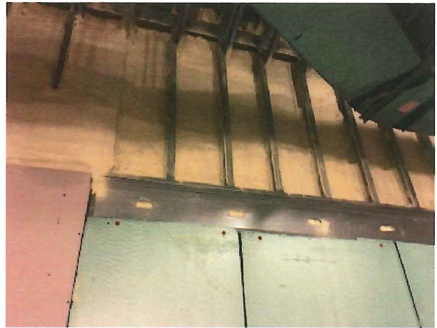
2018.01.30 – Spray insulation needing intumescent paint.
