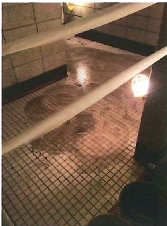
2018.02.15 – Mosaic tile grouting in progress at second floor restroom.
