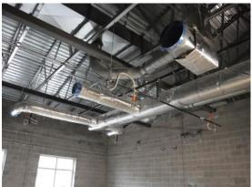
p) Roof deck to block walls in Area B needing to be sealed to prevent air/moisture infiltration into building.
