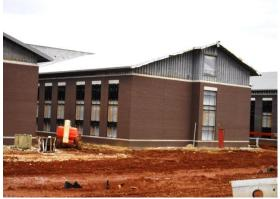
d) Spandrel panels were being installed in the curtainwall at the classroom wing in Area B. The caps for the curtainwall will be installed as the system installation is completed.
