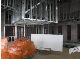
i) Board suspension system is being used for soffits in the Library/Media Center.
