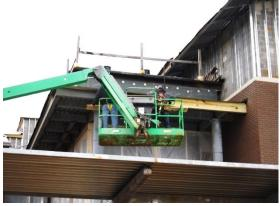
f) Roofers were installing wall flashing material at the expansion joint and exterior walls at Areas A and D.
