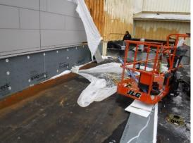
g) Gas cylinder and gutters stored on roof membrane with no protection board.
