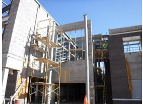
I) The second floor of the main corridor is topped by a high wall that supports steel bar joist and metal deck. When these are in place the built-up roofing can be installed.
