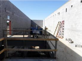
q) Rigid roof insulation was stockpiled on the metal roof deck over the classroom wing in Area B. The roofers were working on the other side of the roof.
