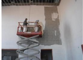
k) The front wall of the Library/Media Center is on place and the steel roof framing is in place ready for metal roof decking. The repairs have been made to the block bearing and the wall at the back of the vestibule. Block pilasters were being added to the side walls.
