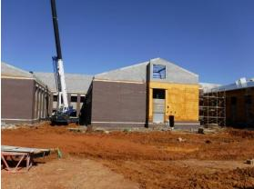
c) Roofers were installing rigid insulation and vapor barrier over the metal deck over the classroom wing in Area B.
