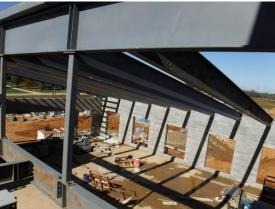
t) Truss bracing at the end of the classroom wing in Area B is in the same plane as the block and does not allow the block to bear on the wall below. I asked Doyle to review this
