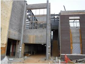
aa) The steel roof joists were being installed over the main corridor. This work is now complete and steel roof decking installation has been started.
