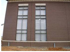
w) The cut brick at the movement joints in the brick look better than they did when they were laid, but there still is a difference in color. The amount of this contrast varies with the direction of the sunlight. The brick supplier needs to review this on site and make a recommendation for correction.
