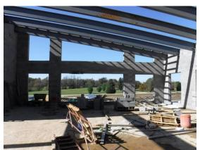
o) Some of the steel framing over the Library has mud clumps that must be removed.
