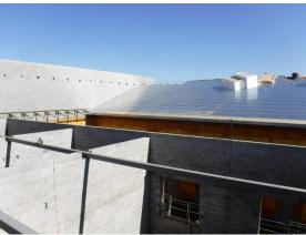
r) The steel framing is on place over the two classroom wings in Area A. These are ready for metal roof trusses.
