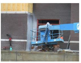
y) The masons were laying the block backup for the screen wall around the exterior mechanical/electrical equipment. The cooling tower is considerably higher than the screen wall. A 4' high guardrail is yet to be installed on top of the cooling tower.
