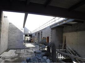
n) The entrance to the Library/Media Center and the steel roof structure are in place. The front wall has high windows to allow ample light into the space. The roof structure is ready for metal roof decking.
