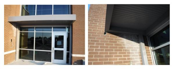
f) The soffit at the entrance has been wrapped with aluminum. The inner vestibule wall and doors still nee to be installed.
