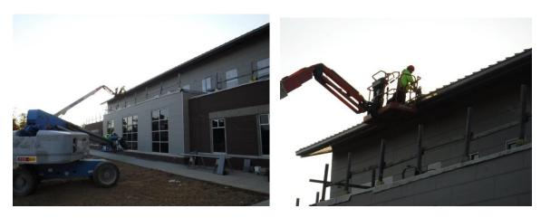
u) The bent plates at the steel frame do not close to the columns. This must be corrected to avoid having a place where birds and insects can enter the soffit at the canopy.
