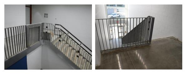
q) Welds on the railings were ground, but primer was not applied.
