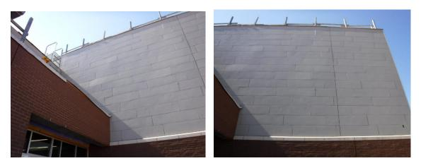
z) The concrete block on the two-story wall in the main lobby is especially rough. This must be corrected.
