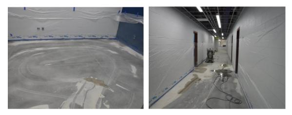
n) The sanding and sealing of the Gym floor cannot be started until the acoustical panels are in place and the electrical work installed.
