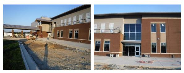
e) The canopy was installed at the entrance at the center of the classrooms. Unfortunately, this was done before the stain was cleaned off the brick. This will now need to be done without damaging the canopy. In addition, the canopy partially covers the back box for a wall mounted light fixture. This may need to be moved.
