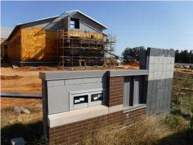
c) The three classroom wings are taking shape. Metal deck is being installed over the rear wing in Area B. Roof framing is in place to receive the trusses over the middle wing and the masonry is being topped out for the front wing.
