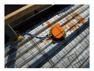
u) The metal roof deck over the classroom wing in Area B can be seen over the middle classroom wing. The seismic wall bracing can be seen running from wall to wall.
