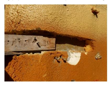
g) The windows on EHMS set back 2" from the face of the brick. The brick returns at the window jambs appear to be adequate to receive the window frames and sealant.
