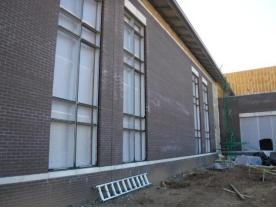
i) The discoloration of the brick at the jambs has decreased since it was laid. I assume that this because the wall has been washed with rain. Too bad, that the brick was cleaned before the window framing was installed.
