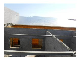
v) The roof framing that will support the metal trusses is in place over the middle classroom wing.
