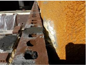
f) Again, all missing spray foam insulation must be repaired before covering with brick.
