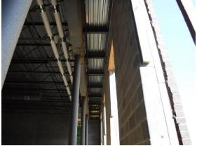
o) The ground faced block under the central stair has lime staining from being in the weather.
