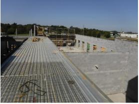
x) The sloped front of the Library/Media Center is defined by the block walls. The roof sheds from the main corridor down to the opposite wall. The front classroom wing is covered with brick.
