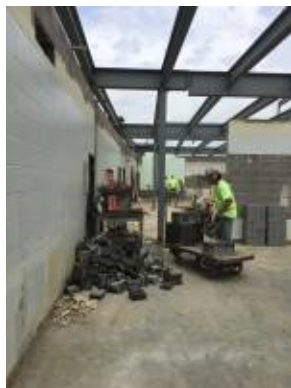
2017.08.31 – Mason cutting block for installation
