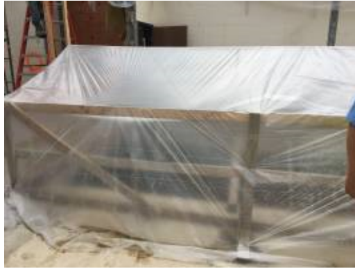
2017.08.31 – Temporary weather protection at excavation to basement
