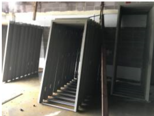
2017.09.14 – Door frames staged for installation
