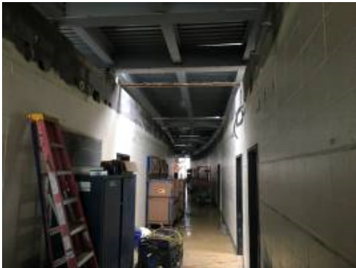
2017.09.14 – Floor deck over existing corridor
