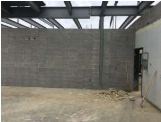
2017.08.31 – Masonry infill at new support column
