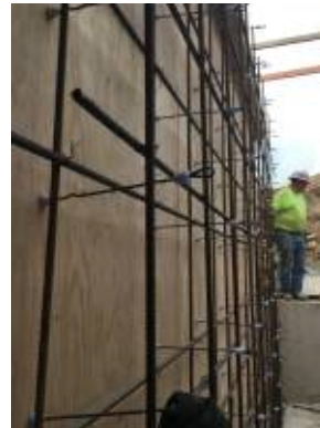
2017.08.31 – formwork and reinforcing at south wall of basement stairs
