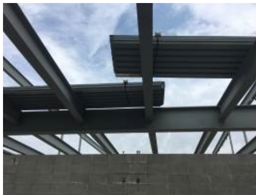
2017.08.31 – Floor deck staged for installation
