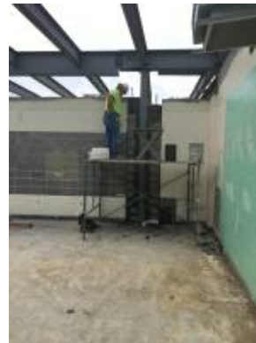
2017.08.31 – Mason installing infill at new support column
