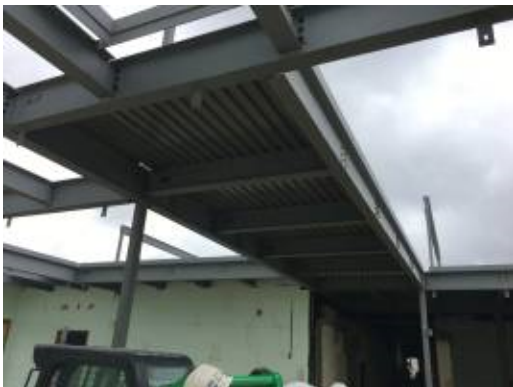
2017.09.14 – Partial floor deck installation above new admin area
