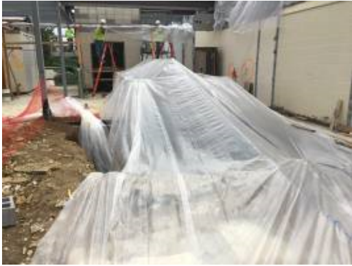
2017.08.31 – Temporary weather protection at excavation to basement
