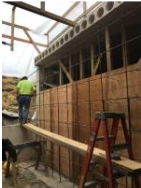
2017.08.31 – formwork and reinforcing at north wall of basement stairs
