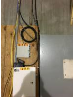
2017.08.01 – Water streaming down wall behind new fiber box
