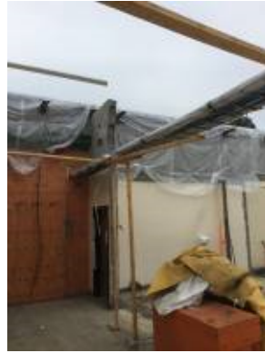
2017.08.01 – Temporary weather barrier north wall of Phase 1
