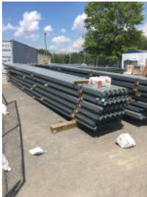
2017.08.10 – Floor deck staged for installation
