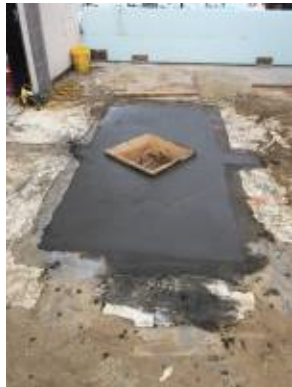
2017.07.13 – recently poured slab at interior classroom pier
