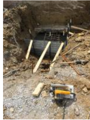
2017.06.29 – underpinning in progress at former cafeteria foundation
