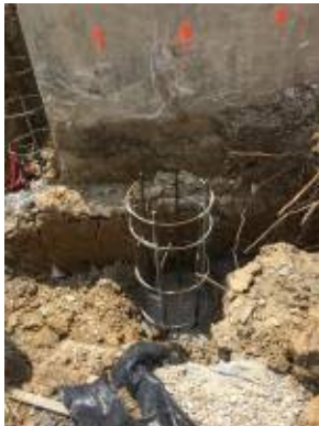
2017.06.29 – Pier partially complete at NE corner of former cafeteria
