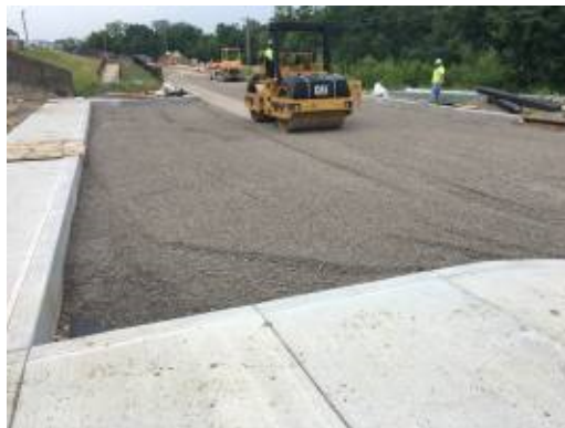
2017.07.13 – rolling base gravel at east drive
