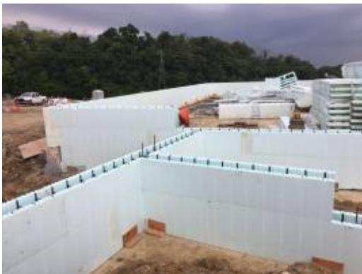
2017.07.13 – ICF formwork and rebar at new entrance
