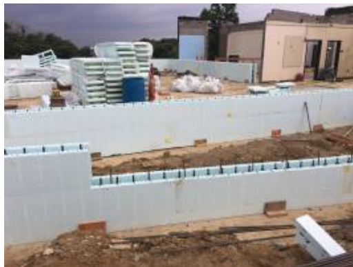
2017.07.13 – ICF formwork and rebar at new entrance
