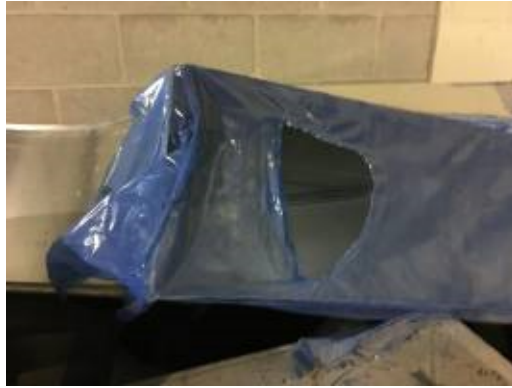
2017.05.18 – Sample of compromised duct wrap.
