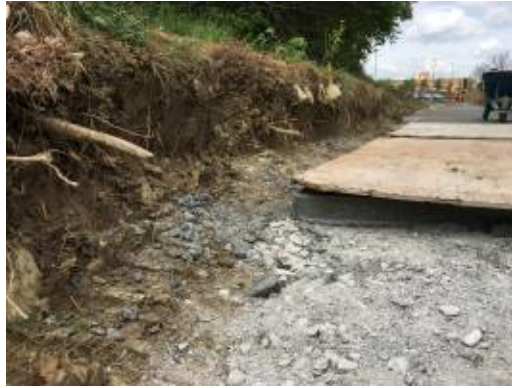
2017.04.20 – Grading issue at new sidewalk and adjacent parcel.
