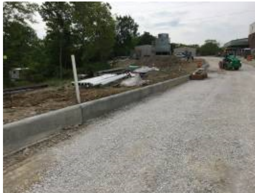
2017.05.18 – DGA being installed along east drive.
