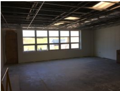
2017.04.12 – Phase 1B classroom with ceiling grid
