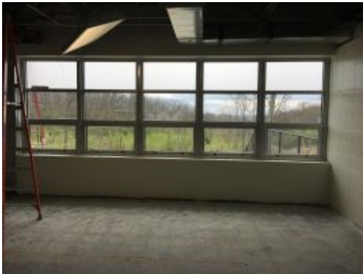
2017.04.03 – Painted Phase 1B classroom
