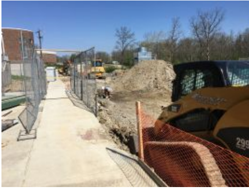
2017.04.12 – Cutting east drive to subgrade
