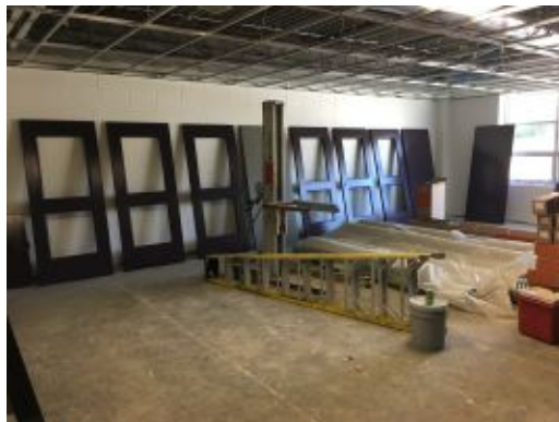
2017.04.12 – Doors being painted
