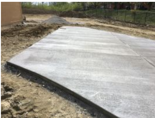
2017.03.30 – Concrete at playground
