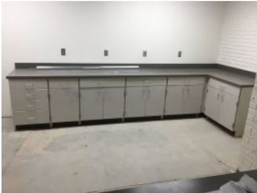
2017.04.12 – Concession stand casework
