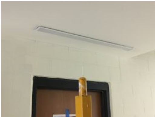
2017.03.30 – Painted hard ceiling outside Gymnasium
