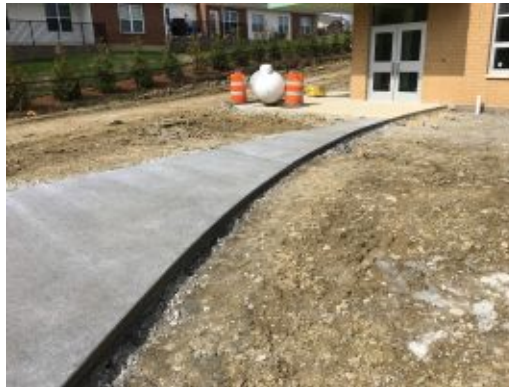
2017.03.30 – Concrete at playground
