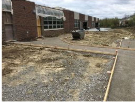
2017.04.03 – Formwork north of preschool playground
