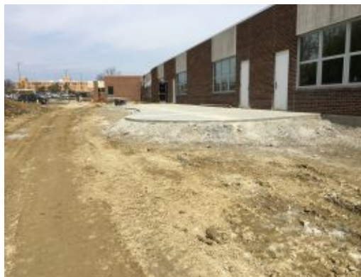
2017.03.30 – Concrete at preschool playground
