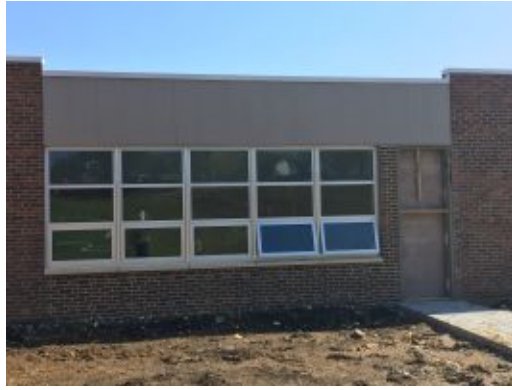
2017.04.12 – Metal siding at Phase 1B classroom
