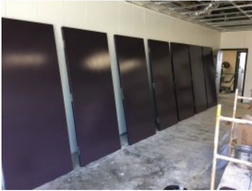
2017.04.12 – Doors being painted
