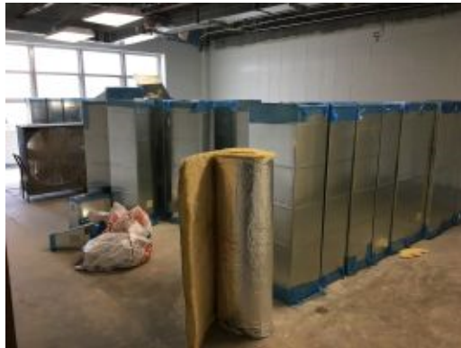
2017.04.03 – Corridor ductwork staged for installation
