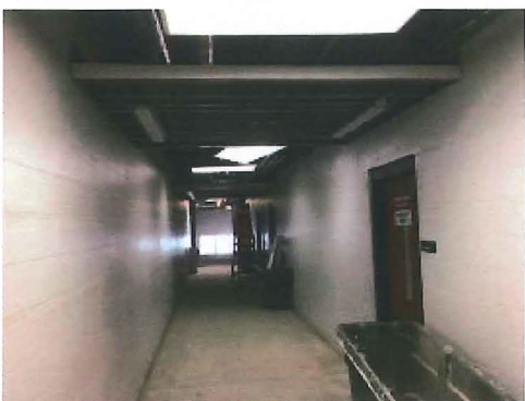
2017.03.13 – Phase 1B corridor hard ceiling framed with light fixtures.
