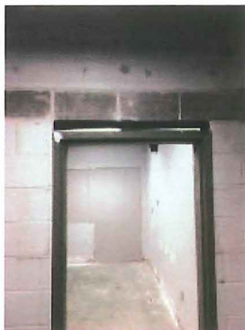
2017.03.02 – Incorrect door frame installed.
