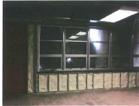
2017.03.13 – Spray insulation Phase 1B classroom.
