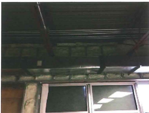
2017.03.13 – Spray insulation Phase 1B classroom.
