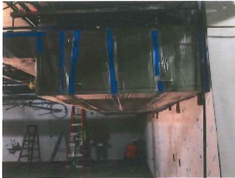
2017.03.02 – Hood with partial stainless steel wall protection installed.
