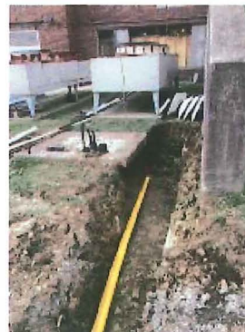
2017.03.13 – Gas service installation near existing chillers.
