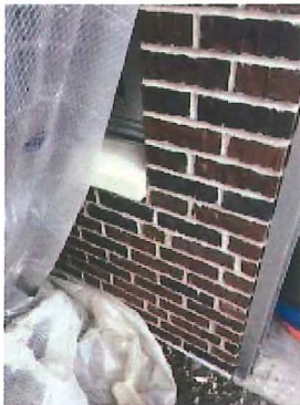
2017.03.02 – Infill brick at a Phase 1B classroom
