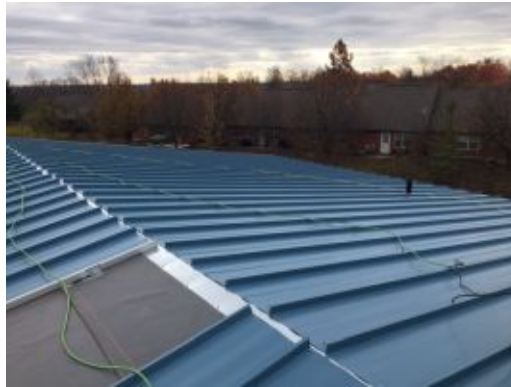
2016.12.01 – Metal roof installation
