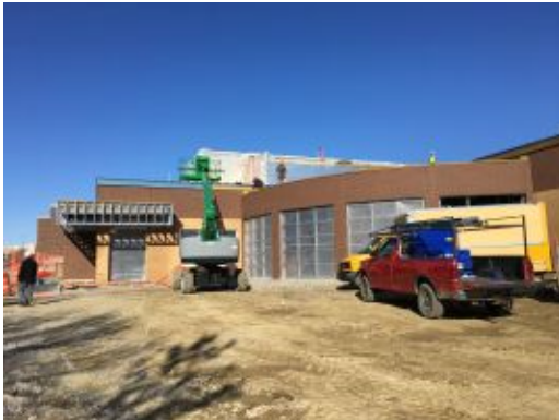
2016.12.08 – Weather enclosure and crew working at platform enclosure above.
