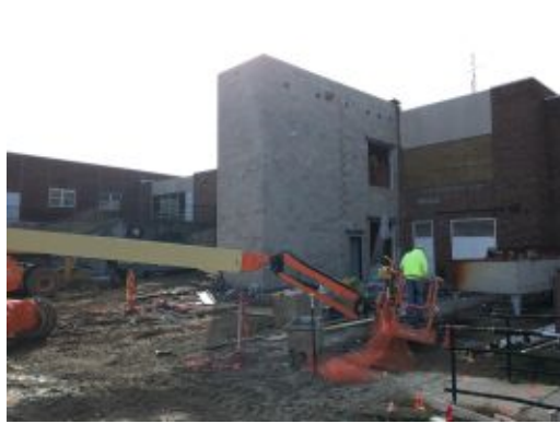
2016.12.05 – Demolition of existing stair tower.
