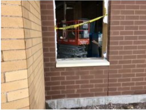
2016.12.05 – Cast sill in place.
