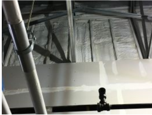
2016.12.08 – Spray foam insulation at truss end wall.
