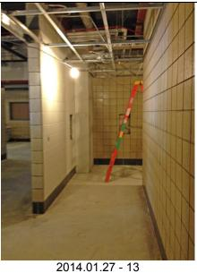
1. First Floor: The structural glazed tile base has been installed in the toilet rooms.
