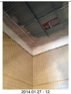
1. First Floor: The intersection between the top of the wall and the roof metal deck has been sealed for fire purposes.
