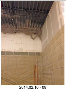
1. Second Floor: The thermal barrier has been installed over the spray foam insulation used at the perimeter joints.
