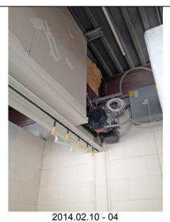
1. First Floor: Installation of the gypsum board infill above the folding partition tracks has been started.
