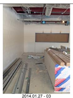
First Floor: Painting of the gypsum board and concrete masonry units is in progress.
