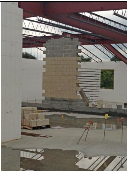
2013.09.16 - 11 1. Installation of roof steel at the west pad.
