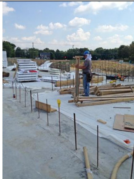
2013.09.09 – 12 1. ICF installation on the second floor of the east pad.
