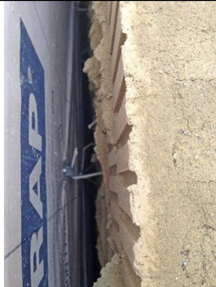
2013.09.16 - 10 1. There were several location where the masonry ties were not properly installed. This has been brought to the attention of the General Contractor..
