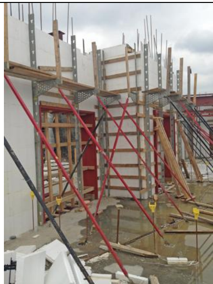
2013.09.16 - 12 1. Installation of ICF at the second floor of the east pad.
