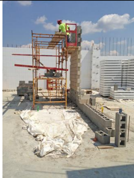
2013.09.09 – 10 1. Installation of interior masonry to support the roof steel at the west building pad - second floor.
