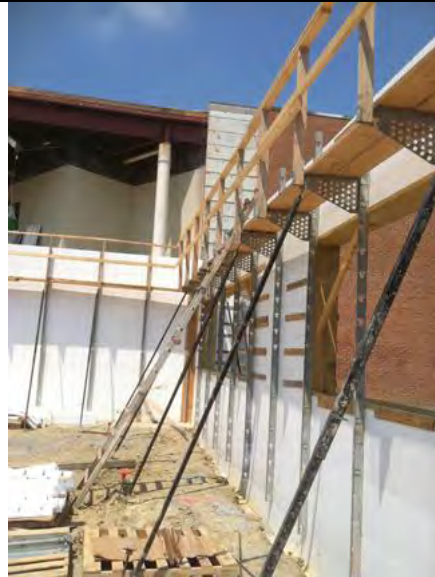
2013.06.26 – 20 1. ICF forms are being installed on the north-west corner of the west side of the addition.
