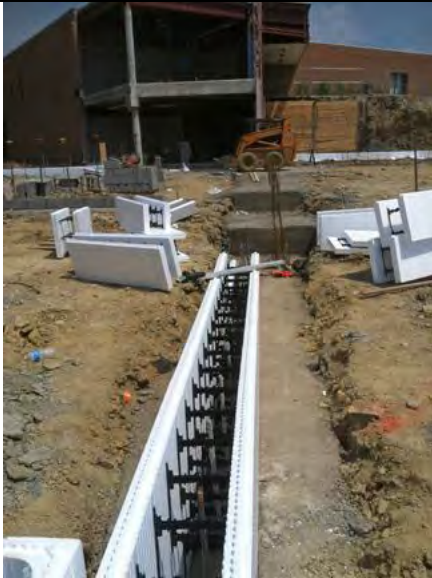
2013.06.26 – 17 1. Installation of the ICF forms.
