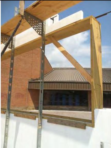
2013.06.26 – 19 1. Openings for windows are being framed along the north wall on the west side of the addition.
