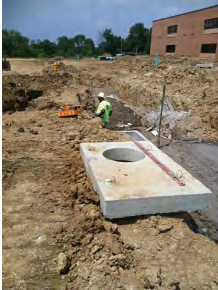
2013.06.26 – 25 1. Installation of storm sewer structures.
