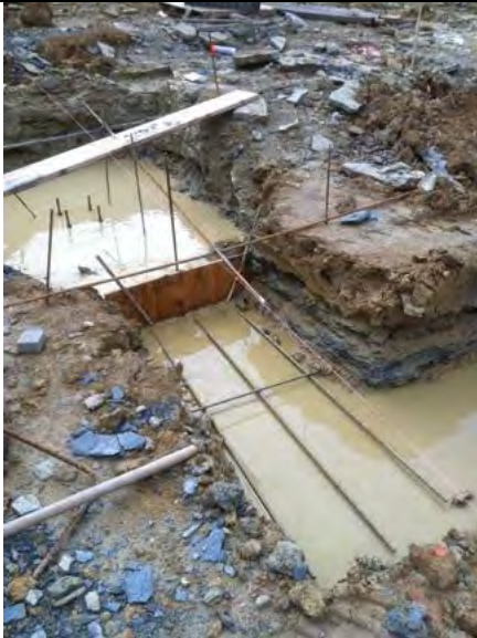
2013.07.02 – 01 1. Excavation for the footings on the east pad continues. Reinforcing is placed in the bottom.
