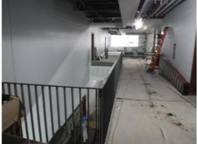
q) The drywall soffit was being hung at the entrance to the student toilets on the second floor.
