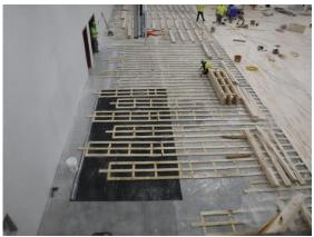
v) The sleeper system is laid over a plastic vapor barrier. The threshold at the entrance will be extended over the expansion space and returned back to the outer edges of the frame.
