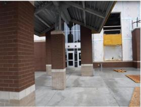
c) Concrete walks are complete at the front of the building. The downspouts are not in place. The plastic weather barrier is in place for the application of the cement panels.
