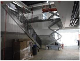
k) The framing for the rear entrance is now in place leaving doors and glass to be installed.
