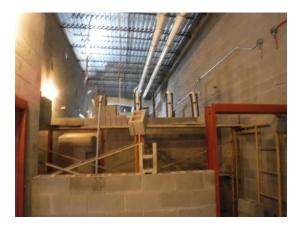
o) Above ceiling rough ins are ongoing in the main corridor on the first floor. Metal stud framing has been installed for drywall soffits.
