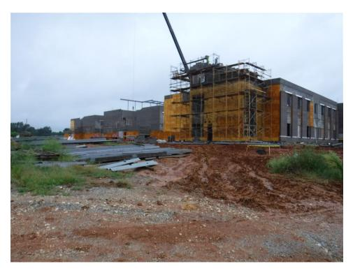
c) The block at the end of the classroom wing will be topped with a concrete cap angled to match the roof slope. Light rain was still falling from the storm during the night, but the masons were continuing to work.
