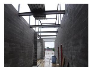
q) The masons are laying block along the secon floor corridor so that the mechanical platforms can be installed over that area and connected to those at the Gym enclosure and to those over the classroom wings.
