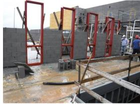
h) The CMU wall at the main entrance has been prepared for the placement of reinforcement according to instructions from Icon.
