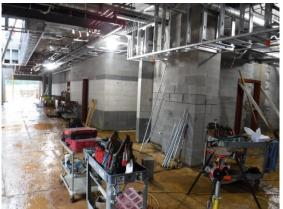
p) The installation of steel framing for the mechanical platform over the middle classroom wing has been started. This framing also provides the bearing for the light gauge trusses that will go over this area.
