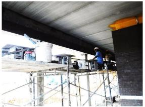
f) The "piers" between the windows at the exterior walls of the Library/Media Center have been laid. Icon has inspected the reinforcement and directed the masons on the placement.
