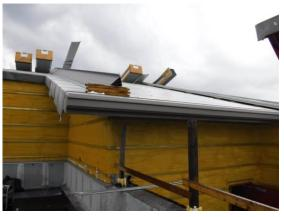
j) Roofers were completing the fascia and gutter at the west end of Area B. Their scaffolding was properly located on plywood protection panels on one side and on the roofing membrane on the other. The hollow metal door and associated hardware to this roof area has been installed.
