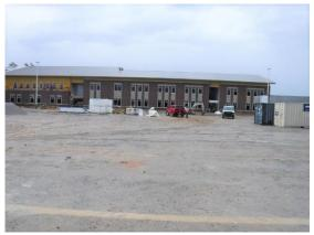
c) Concrete walks have been poured in front of Area C and half of Area B. This provides the base for the aluminum entrances as requested by the window installer. It also provides a place for the water falling out of the gutters to land this preventing mud from splashing on to the brick. This is not the case at the east end of Area C where there is no walk.
