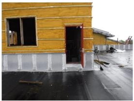
n) The low sloped roof over the front entrance appear to drain well. The door to the mechanical platform is in place. The work ladder to the sloped roof was properly placed on a protection board.
