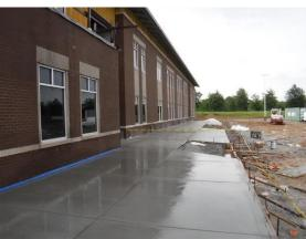
d) The main canopy is complete except for the metal roofing, painting and electrical work.
