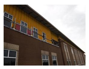
g) The windows have been sealed to the brick. This appears to be a temporary seal that will be covered by the face caps. All joints will need to be completely sealed to the brick. All exposed sealant must be evenly tooled and must provide a finished appearance.
