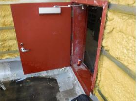
k) It was raining when I took these pictures. There was a considerable amount of water ponding on the roof. It appears that the roof does not slope to the drain sump.
