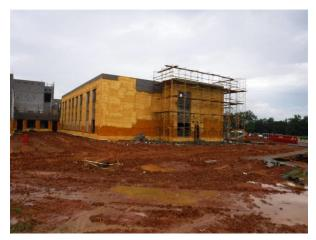
c) Most of the remaining blockwork is at the front of Area A on the second floor including the completion of the classroom wing and the Library/Media Center interior and exterior walls. They were grouting the classroom wing walls while I was on site. I have not heard an update from Doyle about the reconstruction of the piers at the LMC exterior.
