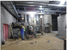
f) The block and slab overpour at the main entrance had been removed in preparation for the installation of the block per the structural detail.
