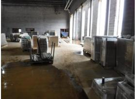
In spite of the rain, the Gym was drier than I have recently seen. Alliance had provided a sump pump shop vacuum and it had removed the water to the lowest level it could pump. There are areas where the floor is completely dry. They had sandbagged the door openings and the roof is now dried in. Very little water was getting in while I was there.
