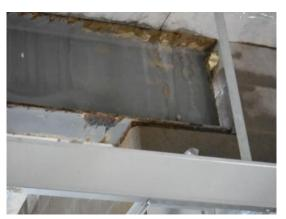
w) Some of the window openings have plastic over wood frames to keep water out of the building. Some of the plastic is torn. A effort must be made to keep these openings sealed an water out of the building.
