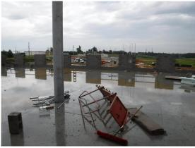
d) Masons had begun laying brick on the back of the Area B classroom wing. They were not present in this area while I was there due to the rain. The brick is almost up to the first floor window heads.
