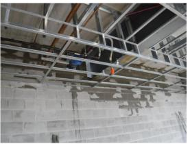
i) In the Progress Meeting, GBMC discussed their proposal to offset and run their piping through the classrooms. Now that the soffit framing is on place, it appears that there is room to run this piping in the soffit. This is being verified by the mechanical contractor.
