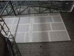
o) Splatters on the ground faced block at the central stair need to be removed.
