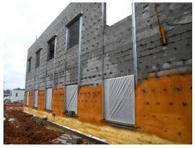
x) There was enough rain that the top layer of the Skudo system was floating on the water. Keeping this system in place in an open building is difficult under the conditions you would expect to have during construction,
