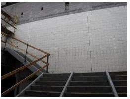
p) The classroom wings are approaching completion. Window closure angles and lintels are in place. The brick below the base flashing has been laid, sprayed insulation is up to the tops of the first floor window openings,
