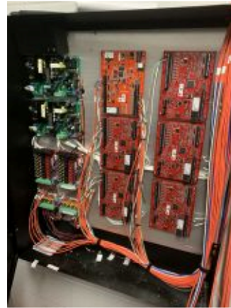
2020.07.14 – River Ridge access control panel
