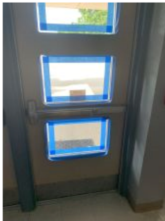
2020.07.14 – Summit View masking for perimeter seal installation at safety film
