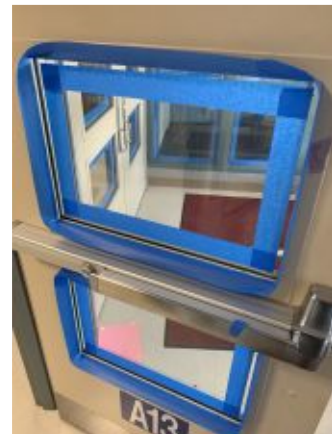
2020.07.14 – Summit View masking for perimeter seal installation at safety film
