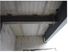
r) Doyle assured me that all of the rust and mud on the structural steel framing will be removed with a wire brush and the primer touched up. That special attention to steel that remains exposed to view after finishes are installed. These surfaces must be prepared for finish painting.
