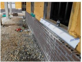
t) The brick cavity at this corner is adequate to allow ventilation of the back of the brick to keep the wall dry. Flashings with properly installed end dams are also critical in keeping water out of the interior of the wall that might migrate to the interior of the building.
