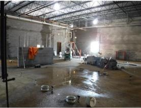
I) The roof trusses that were being installed over Area D during my last visit are now complete. Metal roofing decking was being installed on the trusses while I was on site.
