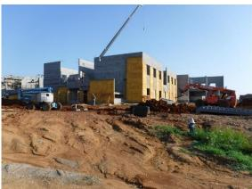
d) It is good to see masons laying block at the resource rooms across the main corridor from the classroom wing in Area B. Laying these walls to bearing height will tie the rear of the building together with full height block.
