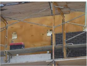
w) The spray insulation also needs to be repaired at the through wall flashings. Before this is done all treaded rods, mortar, loose foam insulation and trash needs to be removed. By the way, the brick in the image to the right is broken and needs to be replaced.
