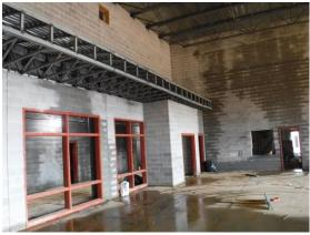
k) Additional rough ins have been installed in the Kitchen. The next step is to add the block walls for the interior spaces.
