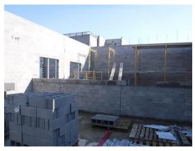
n) Blockwork is being laid for the classroom wings in Area A. Both interior and exterior partitions are being laid.
