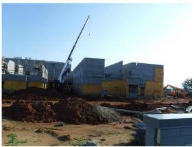
c) At the back of Area B, the walls are extended to truss bearing height except at one bay being used to stock block for the interior partitions still being laid in the area.
