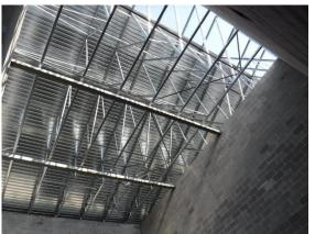
m) The classroom wing in Area B is up to truss bearing height, Most of the interior partitions are in place. Masons were laying block at the remaining interior partitions.
