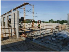
p) The last slab over concrete planks is prepared for the pour the first of next week. This completes the interior concrete slabs for the building except for those on the mezzanines above the corridors.
