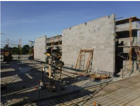
o) The interior and exterior block walls are being laid in the front most classroom wing in Area A.
