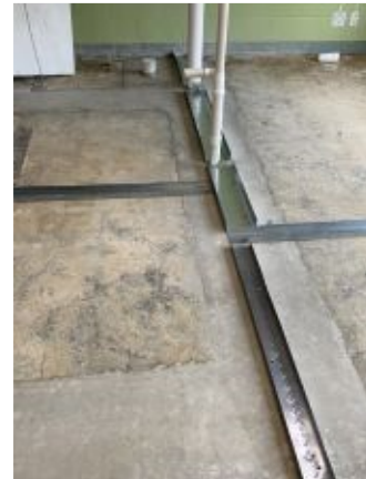
2020.06.09 – Plumbing rough-in through floor track at Ryland
