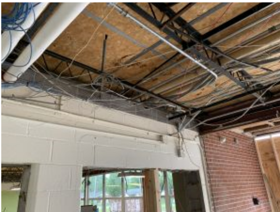
2020.05.21 – Fire barrier at Ryland stops short of deck
