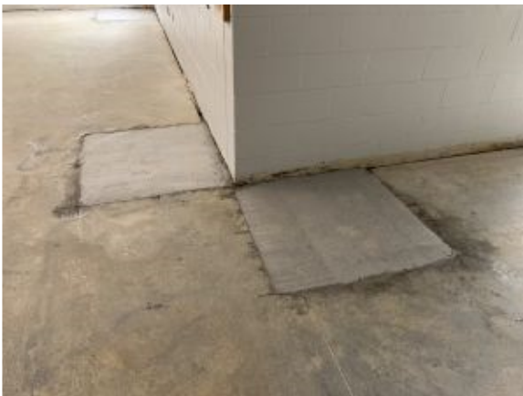
2020.06.09 – Patched slab at interior push pier at River Ridge
