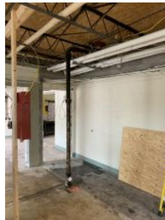
2020.05.21 – Roof drain leader previously concealed in wall at Ryland
