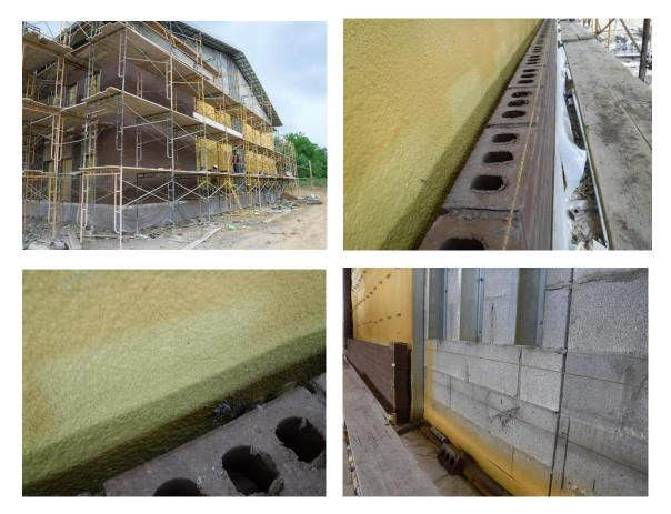
h) Brick had been laid up several courses on the north side of Area C and B on to the Preschool area. It is good to see brick covered to keep water out of the cores where work was not ongoing in this area.
