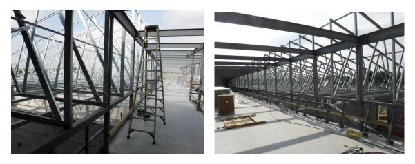
m) Erectors were installing the steel railing around the mechanical platform over Area B.
