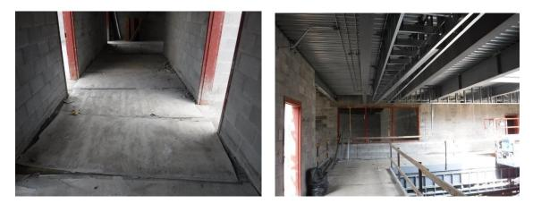
r) The steel roof joists and most of the metal deck are in place over the Gym. Also note that the floor slab is relatively clean. The steel bar joists and metal roof deck are also in place over the Cafeteria.
