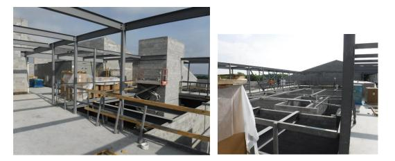
n) The energy recovery unit had been lifted to the mechanical platform level and was sitting in the mechanical room over Area A.
