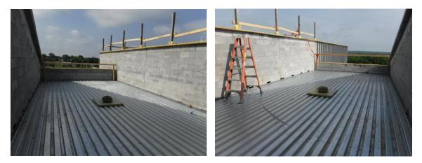
q) Now that the corridors are covered on the second floor, this is a good time to straighten up and retape the Skudo board protection system.
