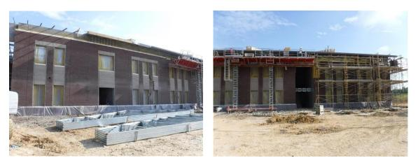
c) After John Stith had questioned the alignment of some of the brick at the windows earlier in the week, the mason had removed the worst of the misaligned brick for realignment. This was confined to one area based on the brick which had been removed.
