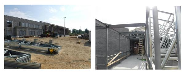
k) The steel framing over Area B has been installed to carry the mechanical platform and the light gauge roof trusses.
