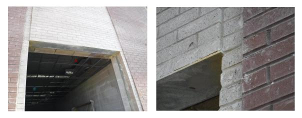
f) Some brick are misaligned in the field panels and will need to be replaced.
