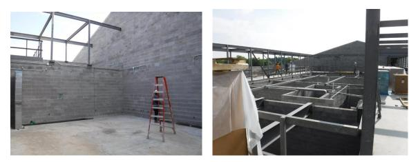
I) Light gauge roof trusses were installed over the front portion of Area B. Gerald reported that the work had been slowed due to a mechanical problem with the crane. It had been repaired.
