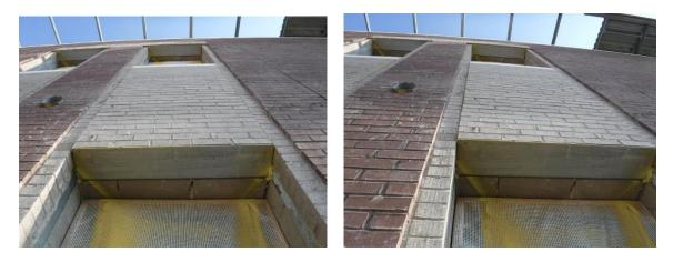
e) Part of the misalignment is caused by the steel lintels over the heads of the window openings. They are bolted to the back of the block at the exterior wall. It is no longer possible to obtain block that is uniform in thickness and plane. Block suppliers reuse their molds thus resulting in the uneven molds and masonry units. The brick panels over the windows were adjusted for these variations in projection and angle.
