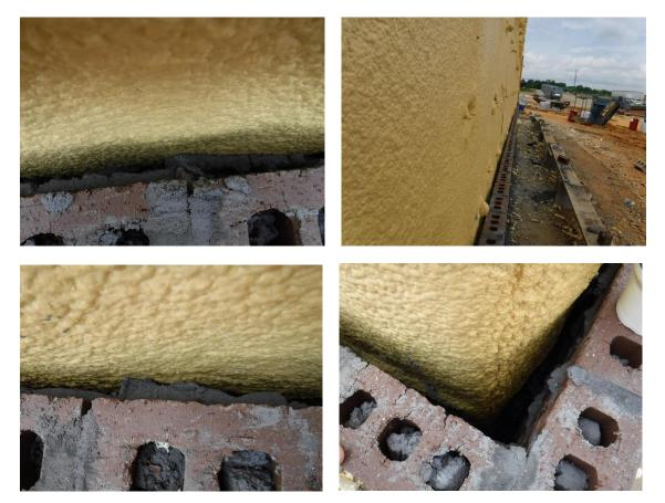
At the front of Area D, the cavity was more open even though it was not the full 1-3/4" in width. It is important that the insulation is on average 3". Some variance is expected due to the nature of the spray foam insulation expanding.
