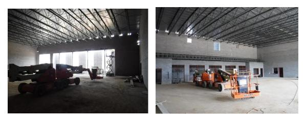
w) Steel bar joists and metal roof decking has been installed over the Kitchen.
