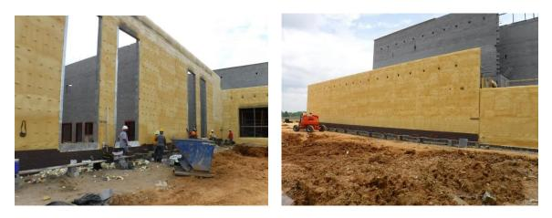
h) The administrative offices are on the first floor of Area A and will be covered with brick. The exterior walls had been sprayed with foam insulation. Metal angles are installed at the window openings to attached the windows and terminate the insulation. The foam is removed to attached the window sill flashing and repaired after the flashing is in place.
