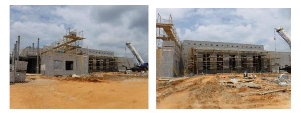
f) To the other side of the Cafeteria, is the Kitchen and loading dock. Beyond that is Area D containing the music rooms. The exterior walls of Area D are being covered with brick over the spray foam insulation. These areas are one story tall allowing the brick to be laid to the full height.
