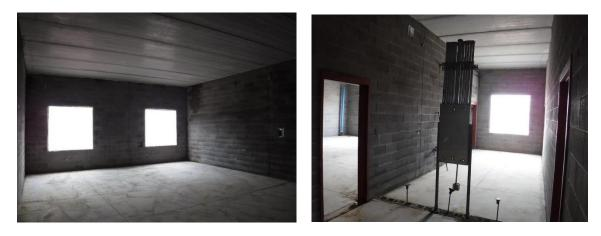
p) The walls for the send floor classroom wing are being laid and include grouted steel reinforcement, hollow metal door frames, plumbing piping and electrical conduits. Openings for ductwork are formed as the block is laid.
