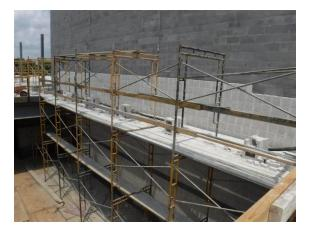
s) The topping slab has been poured over the concrete planks for the classroom wing in Area A that is closest to Area B. The edge form consists of two 2X4's and 2 spacers totaling about 4" in depth. The slab is consistently about ½" below the top of the form. The slab is indicated to be 4" thick on the plans.
