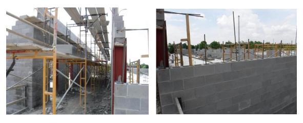
q) Block walls opposite of the classroom wing are being laid up to roof level. These walls tie into the walls at Area C around the Cafeteria.
