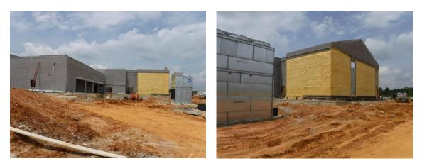
g) Masons were laying brick at the front of Area D for the music rooms. The large opening are windows. The blank wall is the exterior of the PE locker rooms and storage.
