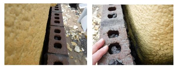
m) As was the case at LTES, the foam insulation had to be removed to attach outriggers to block for string lines and story poles. The mason contractor reported that they will use the same insulation material and sprayer device to make repairs. These repairs need to completely fill the holes in the insulation.
