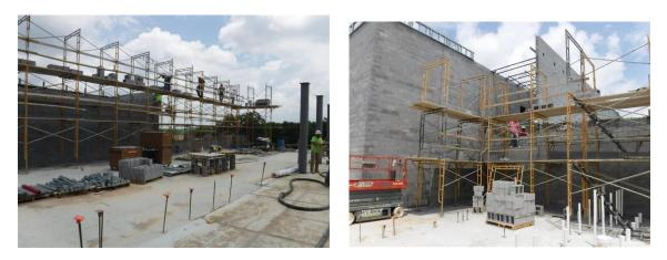
r) Ground faced block is being laid at the Gym/firewall. This is the location of the large open stair in the middle of the building.
