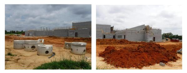
c) From the rear of the site, the window openings on the second floor of Area B are now visible. The exit stair is visible at the end of the wing. The exterior block will be covered with brick.
