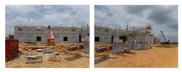
e) From the rear of Area B, the Cafeteria is visible. Masons were laying block in this area to tie Areas B into Area C.
