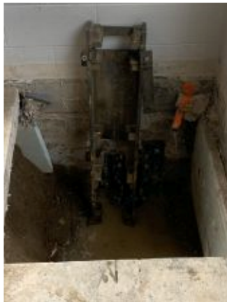
2020.05.14 – River Ridge Media Center push pier installation prep
