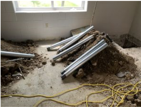
2020.05.14 – River Ridge Media Center push pier sections
