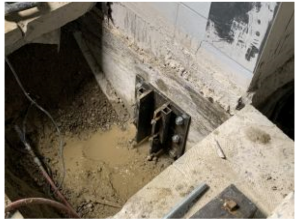
2020.05.14 – River Ridge Media Center push pier bracket
