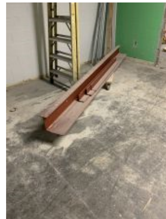
2020.05.14 – River Ridge lintel awaiting installation
