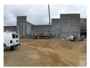
f) The masons were laying block in the Kitchen while working with the plumber to install piping in the walls.
