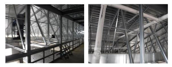
y) There is a significant amount of missing primer on the steel allowing rust to form. The rust must be removed and the primer repainted per the scope in the steel trade contract.
