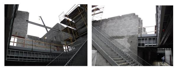
m) The tops of the high walls around the Cafeteria and the Gym are in place. The upper mechanical room is clearly visible from the Gym. Mason helpers were cleaning the bottom of the gym wall where block was laid above.
