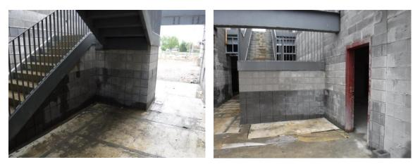
p) Brick was staged at the south wall of Area C. Three courses of brick will be laid. These brick will be below grade and the base flashing. Spray foam insulation will be applied to the exterior block walls above the flashing.
