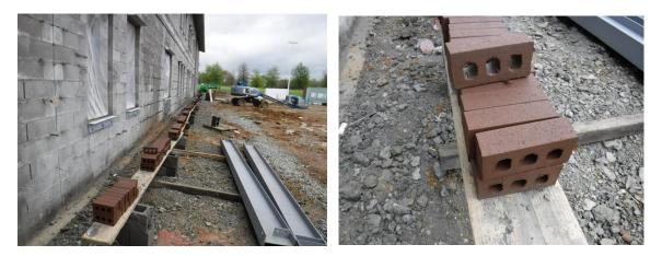
q) The galvanized lintels and sill angles had been installed on the south face of Area C. Refer to the SPIN report for comments on this.
