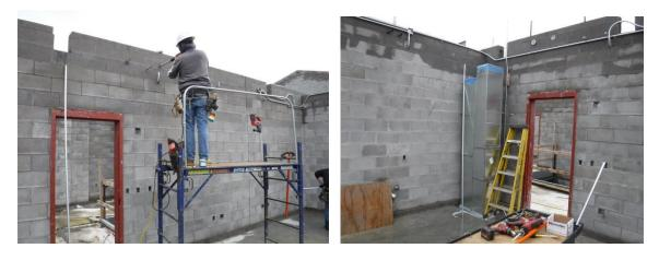
ee) Carpenters were installing pressure treated wood blocking at the window heads over the low roof areas. These areas will receive the fiber cement panels system.
