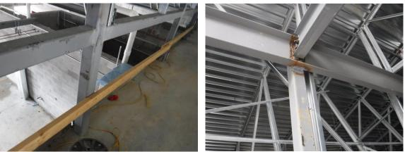
z) The steel framing needs to be cleaned. Mud is visible on some of the members. This must be done before any finish material would be affected by the cleaning process.
