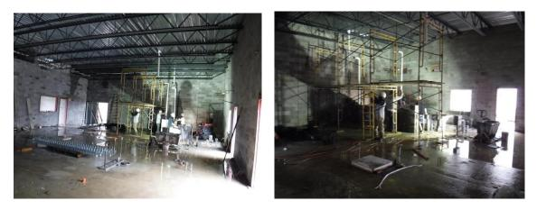
g) Roof deck and joist are in place over the Kitchen and the Loading Dock. When the weather is dry, Gerald plans to have the roof systems installed over these areas. Most of the interior blockwork is in place along the west side of the Kitchen.
