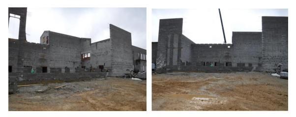
e) As I was leaving, the mason had moved the Hydra-lift scaffolding system into place to lay the rest of the south wall of the Cafeteria.
