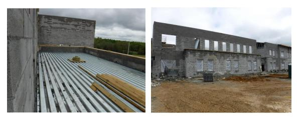
gg) From the mechanical platform, the tops of the classrooms walls in Area B are visible as are the gabled walls at the east side of Area A and the peak of the upper mechanical room wall. The mechanical platform will be installed on the tops of the classroom walls extending it to the upper mechanical room.
