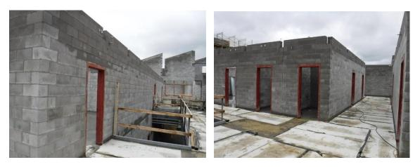
cc) Masons were completing the last of the interior walls on the second floor of Area B. They still need to build block chases around the vertical ductwork in the corners of the rooms.
