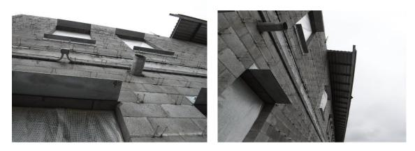
s) If the joints and false joints in the split faced block are not filled with mortar, a considerable amount of repair will need to be made to the damaged block. Most of this is the result of chipped corners.
