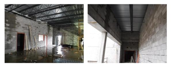
h) Fortunately, the slab construction above the Mechanical Room kept this room with its moisture sensitive electrical equipment dry.
