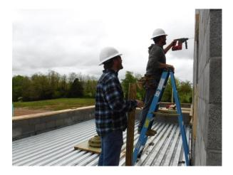
ff) Pressure treated wood blocking has been installed on top the parapets at the low roof areas.
