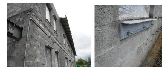
r) The foam insulation will cover all but the eyes on the brick ties. The brick will set on the lintels and a through wall flashing.
