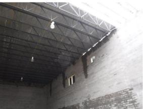
s) The blockwork in the classroom wings in Area A have laid up to plank bearing elevation. The next step will be the placement of steel beams across open areas to support the concrete planks.
