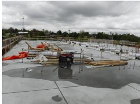
g) The Skudo protection system has been installed over the location for the corridor in the Area B classroom wing. Block has been used to keep the system from being displaced by winds.
