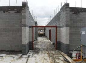
t) The ground faced block with tooled joints look good but additional detailing is required for a finished appearance.
