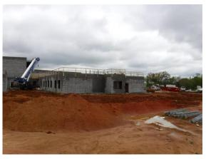
d) Concrete planks are in place at the north side of Area B, ready for the next slab pour. The interior wall in the Resource Rooms was being laid by the masons.
