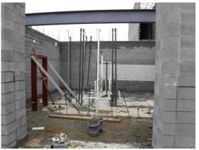
w) The exterior walls around Area A are in place for the first floor. The exterior walls on the west side of Area D will be the next focus for masonry work as the concrete planks and slabs are added to the first floor of Area A.
