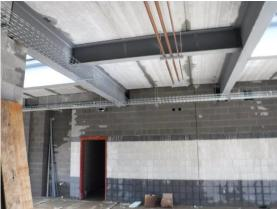
q) The Skudo protection system is over the main corridor. Some of the panels have been displaced and need to be properly located and taped back into place.
