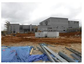
aa) The block walls at the exterior of the Band Room are in place. The sloped beam at the top of the gable that defines the north end of the building needs to be formed and poured.
