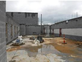
v) Blockwork remains to be laid for the interior toilet walls in Area A and the north-south corridor to the west of the Gym.
