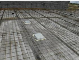
k) Galvanized metal pans have been placed a HVAC penetration locations in the slab. These are capped to reduce the amount of water that can drain to the first floor until the roof is in place over the second floor.
