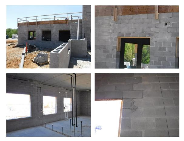
x) Installation of the classroom walls in Area A is critical to the overall schedule. A considerable amount of progress has been made, but much remains to be done. Walls in the east classroom wing are at plank bearing elevation. Walls in the west classroom wing are nearing that elevation. When all of the walls are at plank bearing, the planks are installed, and the slabs poured the walls on the second-floor of Areas A and B can be laid.
