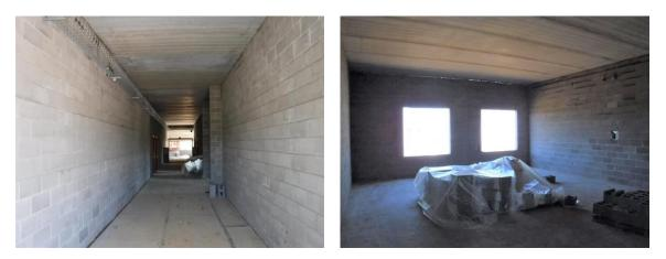
f) Spray foam insulation has been placed in the joint between the tops of the block and the planks to stop cement runs during the slab pour. This material will need to be cut back since it is a flammable and cannot be exposed in the plenum.
