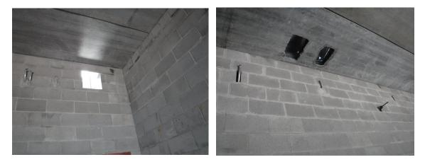
j) The steel beams supporting the planks set on the block walls. In some cases, damaged block may need to be replaced.
