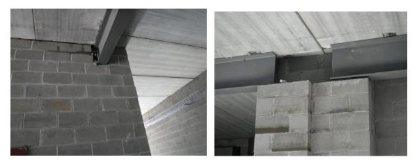
k) Steel framing on steel columns are in place in the main corridor in Area B.
