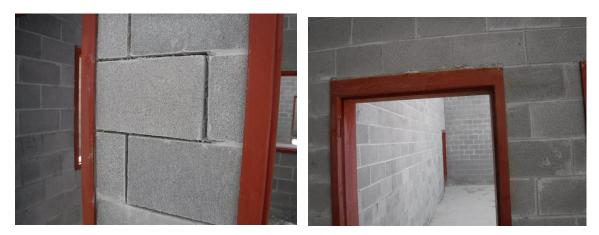
v) Doyle has told the masons that cement matching block textures must be used for repairs to chipped block faces.
