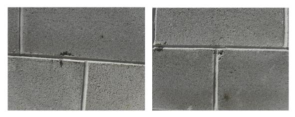
w) The locations where the masonry window openings where corrected are very noticeable especially on the exterior side. Even though these will be covered, the block and mortar joints must be repaired so they provide continuous bearing for the loads above. On the interior, these areas must be repairs so they are indistinguishable from the other block. I am not sure that this is currently the case.
