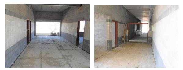
o) The ground faced block at the entries into the Gym looks good. It appears that the control joints above the concrete portals are properly located.
