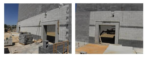
p) The hollow metal frames for the doors and windows into the Cafeteria are in place for block after the walls are laid in Area A and D.
