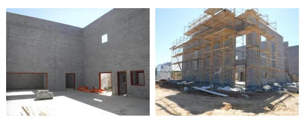
u) Masonry repair work is ongoing. Mortar drips need to be removed from hollow metal frames.
