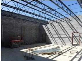
k) The masons continue to complete the tallest walls around the mechanical platform between the Gym and the Cafeteria.
