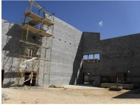
I) The concrete beam supporting the block above the loading dock and the concrete dock are in place. Supporting steel and the roof deck and roofing will installed next.
