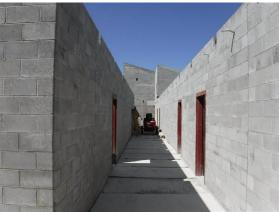
e) The elevator shaft is being laid above the second-floor level. It will need to be capped before the roof trusses area installed. The carpenters need to erect a barrier at the opening.
