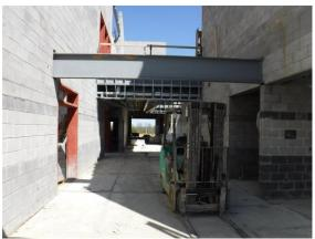
z) Until the building is dried in, we will continue to see staining of the masonry. When the walls are dry, these stains need to be completely removed so the paint finish is not affected.
