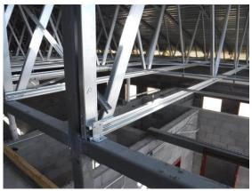
s) Steel tube seismic bracing connects the tops of the walls above Area C. Where the primer has been scraped, the rust needs to be removed with a wire brush and touch up primer applied.
