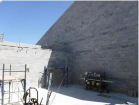
h) Plumbing rough-ins have been installed ahead of blockwork in Area B.
