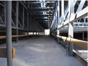
q) Most of the roof decking is in place over Area C except at the east end. The light gauge metal trusses are in place and generally appear to be straight. The roofer needs to evaluate the roof deck for it providing a proper substrate for the metal roofing.
