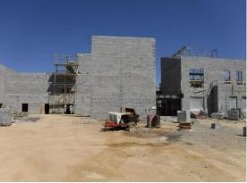
c) The concrete crew had formed and poured the raked beam at the east end of Area B and at the east wall of the Cafeteria.
