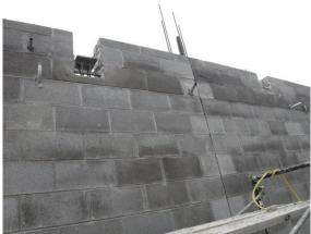
g) The interior block walls for the second floor of Area C are in place. The electrician has installed conduits on the walls and has pulled wire in some cases.
