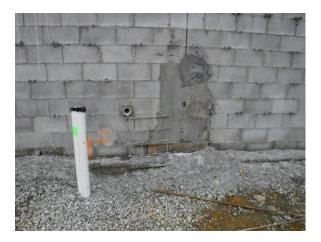
s) The ground faced block and regular block that out of plane at the center stair was being removed in preparation for the repair to straighten this wall.
