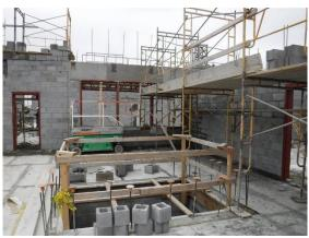
k) Steel roof deck and joists has been placed at the north end of the Library/Media Center. This allows for the completion of the framing for the soffits in the Library/Media Center and rough ins below the roof area.
