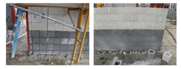
d) The outside corners of the ground faced block have bullnoses as specified. These block cost about \$40 each. The mason is being extra careful to not damage these blocks.
