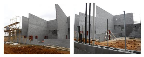
n) Doyle noted that the use of the Hydro Lift scaffolding system has accelerated the blockwork in areas where it can be used. These are typically long walls that benefit from the long spans and supports the system employs.
