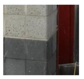
e) The concrete block fire wall around the Gym and extending in front of the Cafeteria consists of two independent block walls. The wall ties sticking out of the Gym wall would tie these two walls together so they do not act independently. The ties will be removed and two courses of block will be cut free from the Gym wall.
