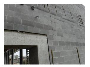
g) Doyle said that the dark mortar can be successfully cleaned off of the ground faced block. It is important that the mortar not be left to harden in the block faces so the joint appears as a smear instead of a clean line just in the joint.
