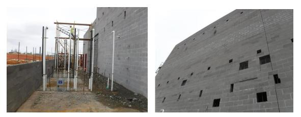
m) Blockwork in Area D has been extended up to truss bearing height. Some of the trusses in the area bear on steel framing supported by columns above the mechanical mezzanine.
