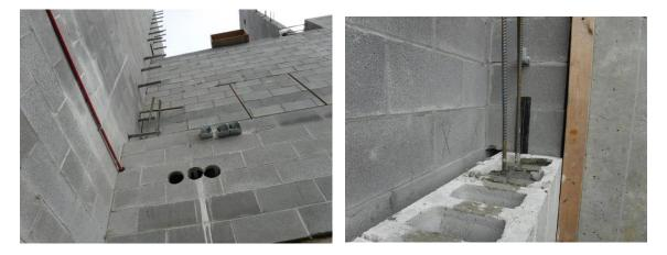
f) Concrete block wall over the concrete portals at the fire wall, do not bear on the portals. The control joint at the end of the bond beam must be on the wall side of the portal.
