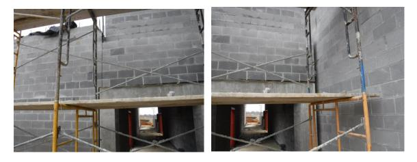
i) Masons were reworking the exterior walls at the east side of Area B where the window openings were laid as if the windows would be two stories high. The block at the jambs has been cut back to reveal the grouted cells. JRA, Solid Ground and Icon have noted this discrepancy in their reports. The corrective measures cited was to remove the upper portion of the block and reinforcing to restore the wall to the original design intent.
