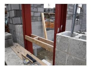
r) Overall, a significant amount of blockwork has been installed. The addition of the steel framing and the precast concrete planks for the second floor of the classroom wing will allow for the completion of the walls.
