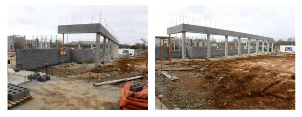
I) The exterior block wall at the west side of the Gym has been started. The wall along the corridor and above the mezzanine is laid to roof joist bearing height. Openings in the wall are for mechanical penetrations from the mechanical mezzanine.
