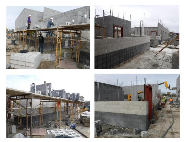
c) The ground faced block needs to b cleaned and sealed. Overall the work is acceptable thus far. Block the block joints and the false joints have been filled with mortar and tooled with a concave joint. The joints at Lincoln Trail Elementary School are struck for the block joints and the false joints are left open.
