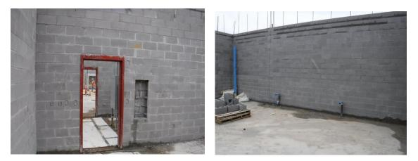
q) Doyle noted that one of the door frames was scheduled to fit into an 8" concrete block wall but the wall is 12" wide at that point. JRA agreed that the frame could be located in the center of the wall so that the work could proceed. The base at the returns needs to be anchored to the bullnose corners so that it does not separate over time.
