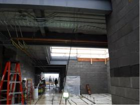
q) Due to the excessive amount of rain, water from the second floor slabs is being directed into the floor areas and the block walls on the first floor. This is causing staining elements in the block to leach out. These will need to be cleaned when the building in enclosed.
