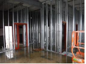
m) Detailing of the metal studs around the hollow metal frames at the slab appears to be per the specifications. Double studs were used at jambs. A check of the frames, demonstrated that they were rigidly in place. Slip track was used at top of studs.
