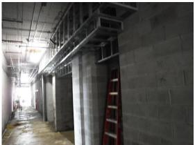
p) The floor opening and cross corridor beams are in place at the lobby and south to north corridor.
