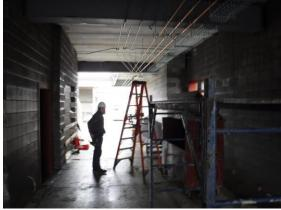
u) The steel stairs and railings are in place in Area B. Since they are exposed to the elements until the roof is in place, these need to be monitored for rust. Missing primer needs to be replaced and any rust that is discovered needs to be removed as soon as possible.
