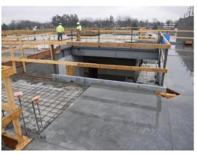
Floor openings at the second floor were framed with steel tubes. The topping slabs will e) pour to the steel.
