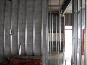
o) Metal stud soffits were being installed at the entrances to the Toilets in Area B. Other soffits had already been installed.
