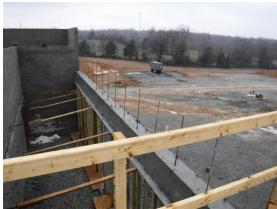
i) As the second floor slabs are completed, the steel bar joists have been put into place for the roof area that covers the first floor.
