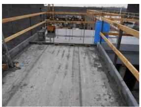
Steel diamonds were in place at the topping slab edges from the previous pours. f)
