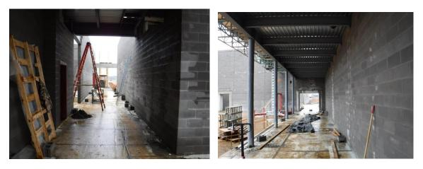
p) The plumber has installed their rough ins ahead of the block walls. The high winds the night before had knocked one of these down. The electrician has prefabricated his wall box/conduits to place in the block walls as they are laid.
