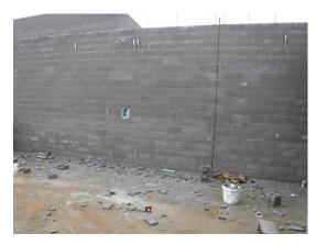
e) Concrete block walls were being laid to the south of the fire wall for the Low Incidence Classroom.
