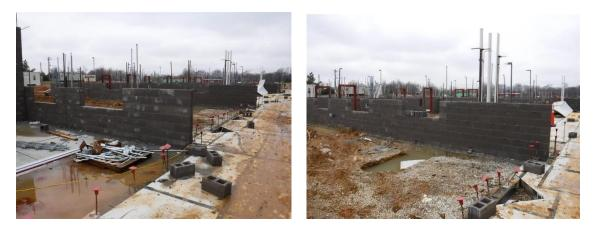
g) The top layer of the Skudo protection board had blown up from the high winds experienced the night before. Doyle said that he had contacted Wittenberg to return to the site to make repairs. This occurred in spite of having concrete block located on the system.
