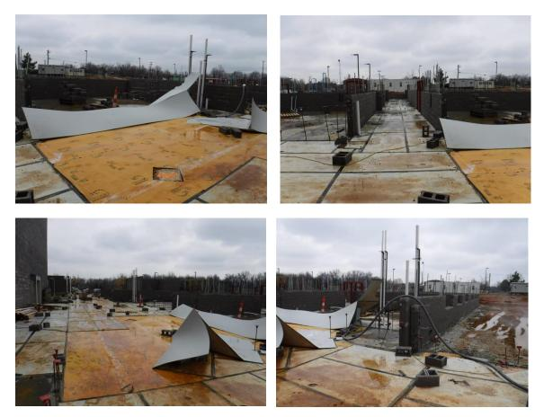
h) The south wall of the cafeteria and some of the walls in Area B have been laid up to bearing elevation.
