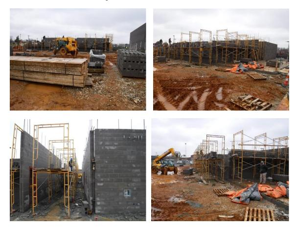
c) As the Classroom walls are being laid, the data/power boxes for the TV monitors and the teacher's stations are being placed in the walls. The location of the teacher's station box is affected by the window location. In one case, the box is to the left side of the window to avoid having it too close to the corner of the room. Doyle said the locations of the boxes have been coordinated with HCS.
