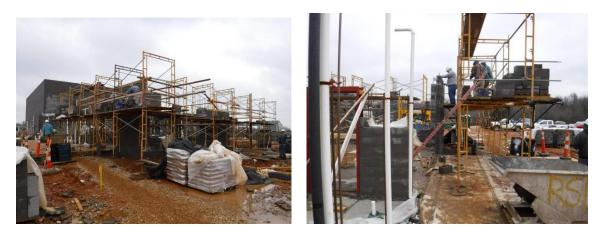
f) Concrete block walls had been laid up to the first grout lift for the Classroom walls in Area A.
