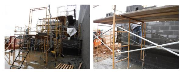
m) The masons are using Hydrolifts for the high walls above mezzanine.
