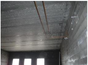
m) The general trades contractor was going to remove the water ponding on the classroom floors. The Skudo system traps the water at the doorways thus causing about ½" of water to be trapped in the rooms.
