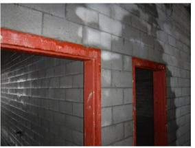
h) The toilet on the east-west corridor is enclosed with block. The precast concrete planks will span over the top. Then the interior block walls will be laid.
