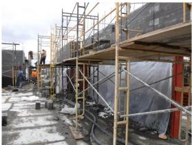
e) The ground face block looks good, but still needs to be detailed and sealed. The outside corners of the ground face block do not have the bullnose radii that occurs on the block above them. A grinder with a built-in radius will be used on the ground face block to match the bullnose on the block above. This must provide a finished appearance.
