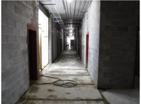
I) After the heavy rain on Sunday, the walls and ceilings of the rooms were saturated with moisture. This partially the result of the water that is ponding on the floors.
