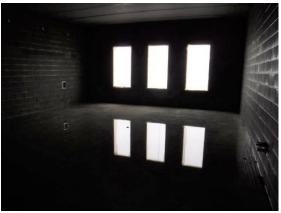
n) Where the moisture has saturated the block walls, lime was wicking out of the block. This needs to cleaned off of the block as the it is detailed.
