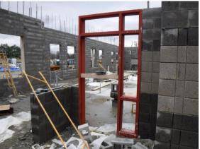
f) The ground face block needs to be cleaned. The joints need to be tooled per the approved sample. If edges and corners need repair, this must be done to match the surrounding units.
