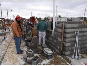
g) The general trades crew had set hollow metal door frames ahead of the masons laying block walls. The frames were being checked for plumb as the walls were being laid.
