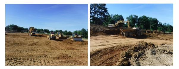
i) Blake has reported some soils did not meet the compaction requirements on the initial pass and had to be ripped and reworked to achieve proper compaction.
