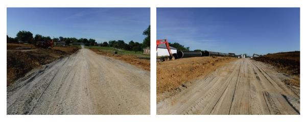
n) The service road to the north of the building has been graded and covered with crushed stone.
