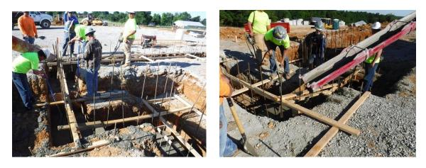
e) The footings have the proper keyways at the ends of pours and the dowel spacing appears to be as indicated. Concrete brick was used to elevate the bottom rows of reinforcing steel off of the bottoms of the excavations. Refer to the SPIN report for dowel placement, spacing and size confirmation.
