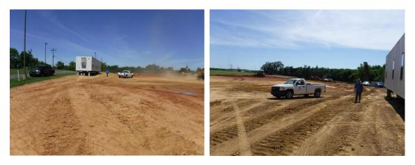
c) The soils materials were relatively dry and workable. Rain is predicted over the weekend. Dickie said the excavator will seal the pad before the end of the day so that the rain will have a reduced impact on the material.
