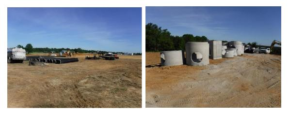
k) The storm line was being laid down the hill to the headwall outfall structure into the natural swale to the north of the site. The excavator reported hitting some rock that he removed with a hoe ram.
