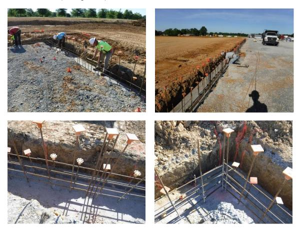
d) Concrete footings were being poured. Solid Ground's field technician was retrieving concrete for cylinders. Blake reported that the concrete from the Elizabethtown IMI plan was of good quality with proper slump, density and compression rating when tested.
