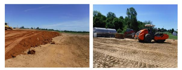
d) Dickie reported that the excavators are using laser guided equipment to insure the placement of fill in lifts as required by the specifications. Thus far, the compaction reports have been within the specifications.
