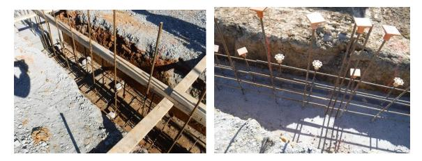
f) Reinforcing steel is stockpiled on site. Footing matts are being prefabricated for insertion to footing excavations.
