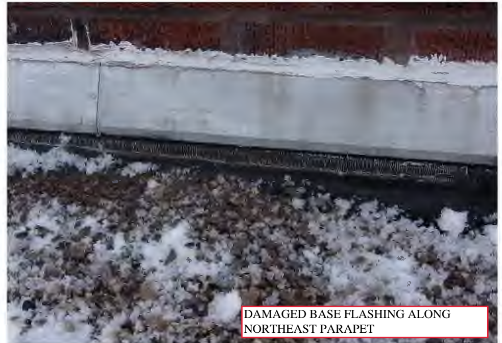
DAMAGED BASE FLASHING ALONG NORTHEAST PARAPET (SEE AERIAL MAP)
