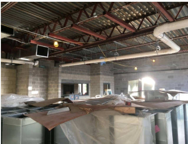
2018.10.09 – Roof overflow pipe installed.
