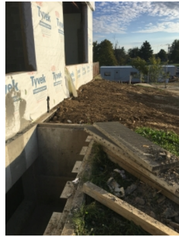
2018.10.09 – Backfill along south wall.
