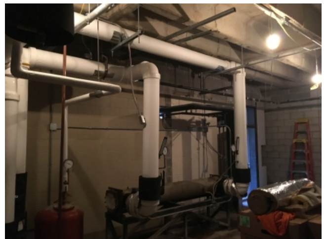
2018.10.09 – Insulated piping at Beechgrove chiller barrel.
