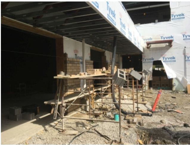
2018.10.11 – Brick installation at courtyard.
