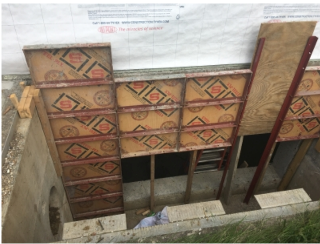
2018.10.02 – Formwork at area well infill.
