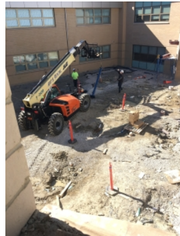
2018.10.23 – Shade canopy column being installed.
