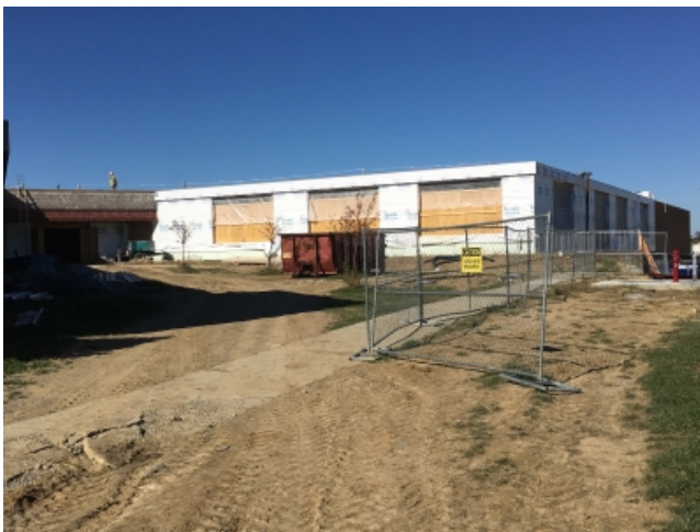
2018.10.23 – Temporary infill at window openings.
