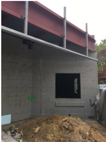
2018.09.10 – Support framing for the cast stone over the entry has been installed.
