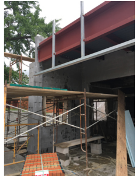
2018.09.10 – Support framing for the cast stone over the entry has been installed.
