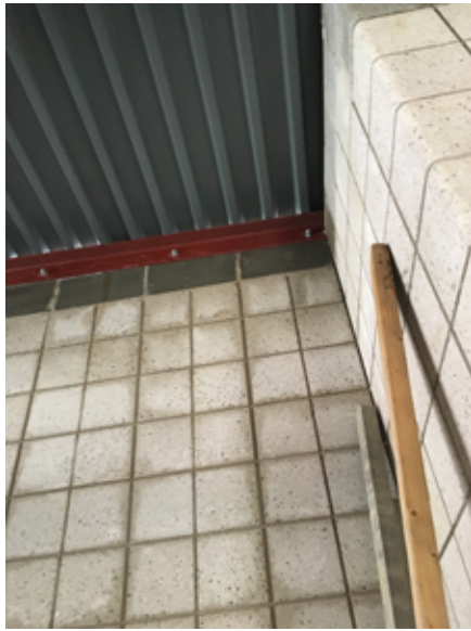
2018.09.10 – View of roof deck and perimeter support angle.
