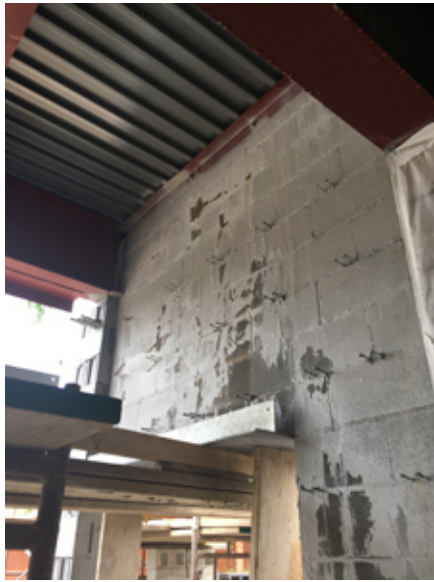
2018.09.10 – The second coat of the air and moisture barrier washed off due to a sudden rain. The contractor stated this would be recoated.
