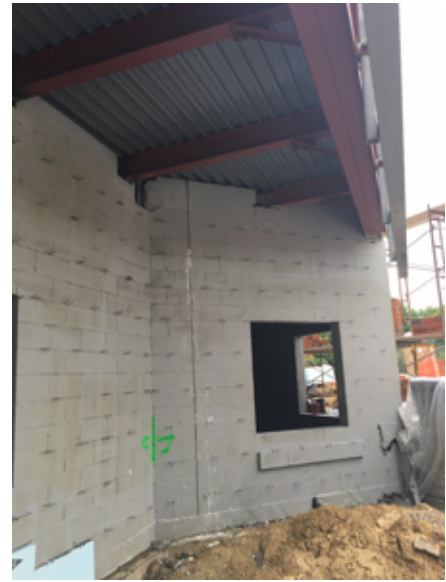
2018.09.10 – The exterior concrete masonry units were coated a second time with the air and moisture barrier after it was determined the initial coating was too thin.
