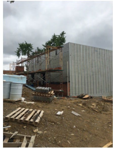
2018.09.10 – Metal furring has been installed for the prefinished metal siding.
