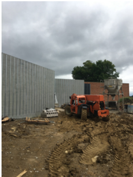
2018.09.10 – Metal furring has been installed for the prefinished metal siding.
